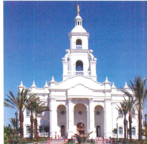
Latter Day Saints Tijuana Temple Category: International Buildings Structure Location: Tijuana, Mex. Architect: CRSA Engineer of Record: ARW Engineers Precast Producer: Willis Construction Company, Inc. Photo: Roland Byers/Willis Construction Inc.
