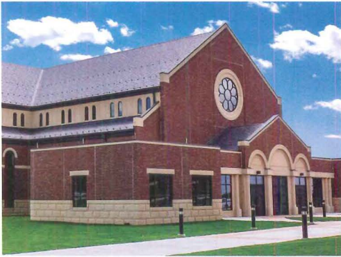
St. Mary Catholic Church and School Category: Schools (K-12) Location: Joplin, Mis. Architect: RDG Architects Engineer of Record: Thompson, Dressen & Dorner, Inc. Precast Producer: Enterprise Precast, Inc. Photo: Julia Phillips Photography and Enterprise Precast Concrete Inc.
