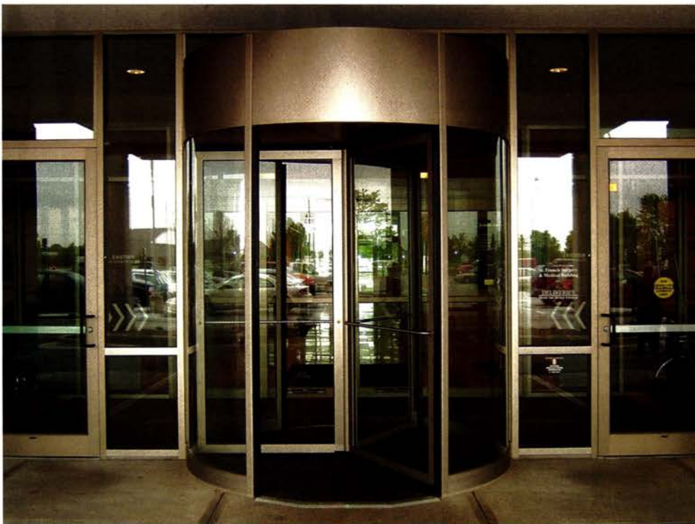
For a clean look, architects can specify stainless steel or other type of metal.
