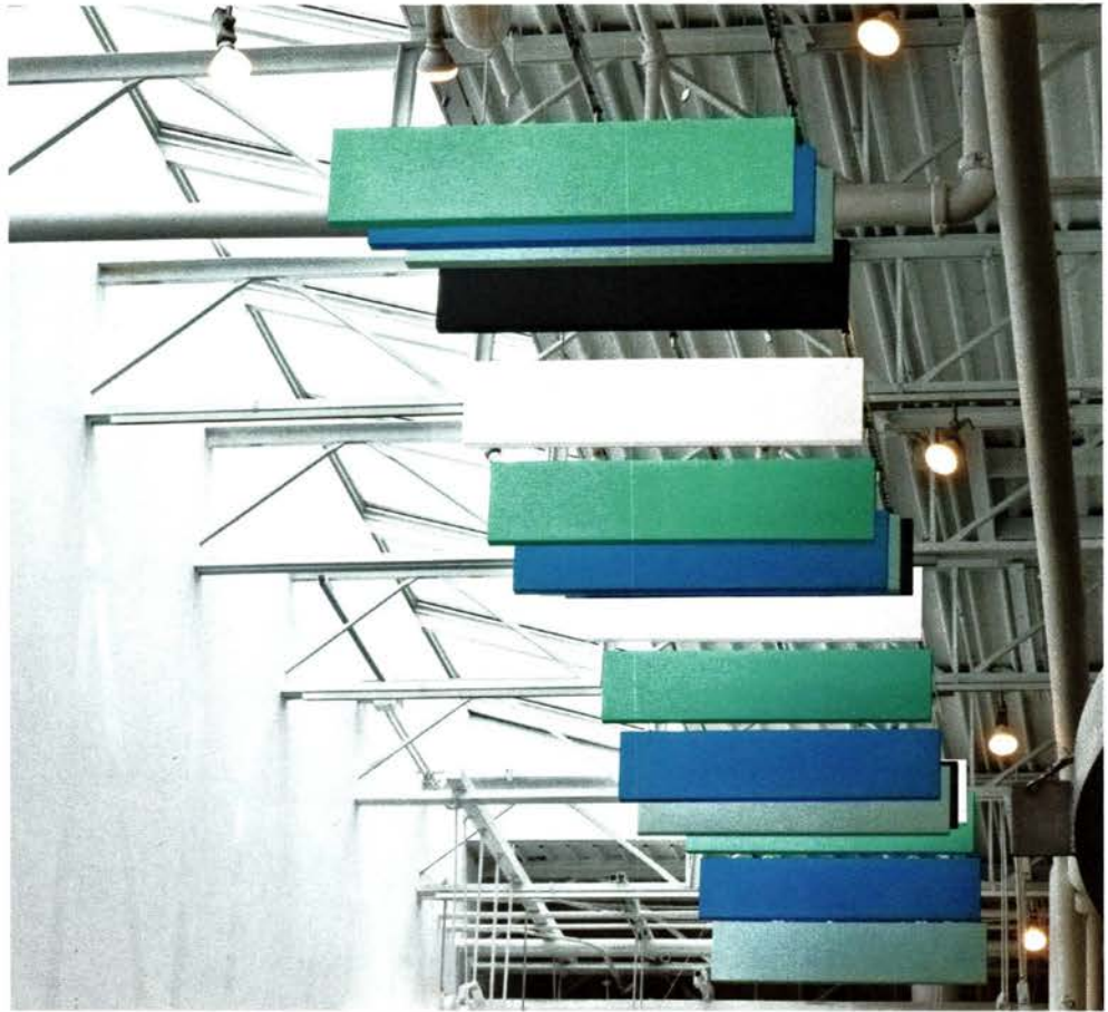
Left: Sound reverberation can be controlled with ceiling systems that are both acoustically efficient and visually exciting. Right: Vertical acoustical treatments such as baffles used in this ceiling space help to control reverberation time and overall sound quality.
