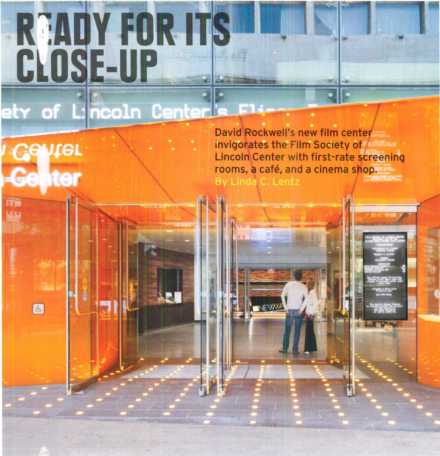
ABOVE: The new film center fronts West Sixty-fifth Street with a vivid orange marquee, an LED carpet, and a welcoming transparency that reveals its community-friendly public areas as well as the central amphitheater, directly beyond.
