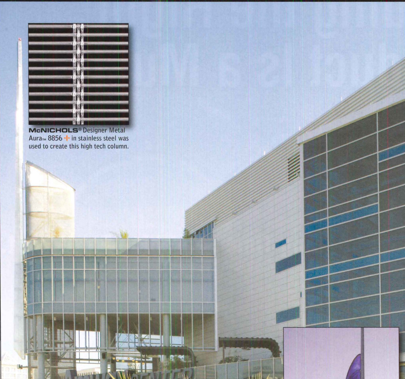
The Amway Center's 180-foot needle tower is a beacon in the city of Orlando. The column is made of McNICHOLS® Designer Metal - Aura™ 8856 + in stainless steel.
