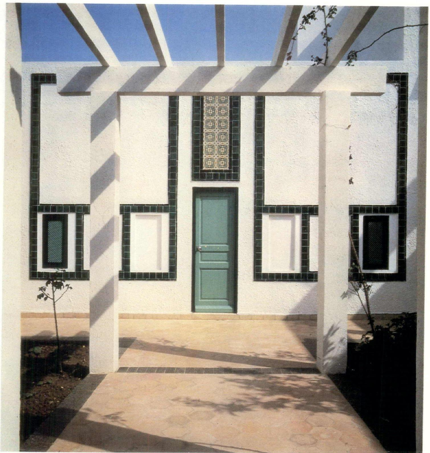
Bands of traditional tiles surround windows and form simple geometric patterns, not unlike those to be found on courtyard walls in traditional Arab houses. The windows are small and protected by wooden screens that filter the light. Doors are all of wood painted light green with dark-green frames. All joinery has been done by traditional methods.
