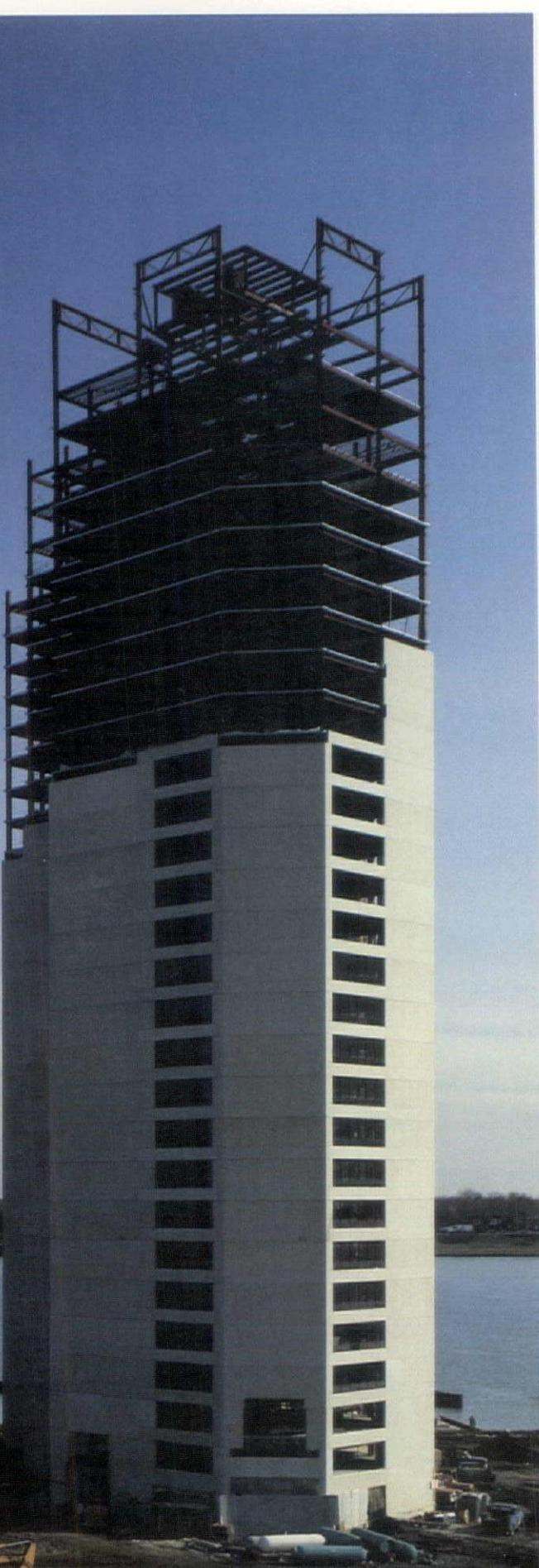
After carefully evaluating the costs of traditional systems including composite design structural steel and reinforced concrete, the designers and builders of the Riverfront Apartments in Detroit chose an innovative alternative in high-rise structural design. By using Vulcraft steel joists, the construction of the 29-story twin towers stayed on time and on budget.
