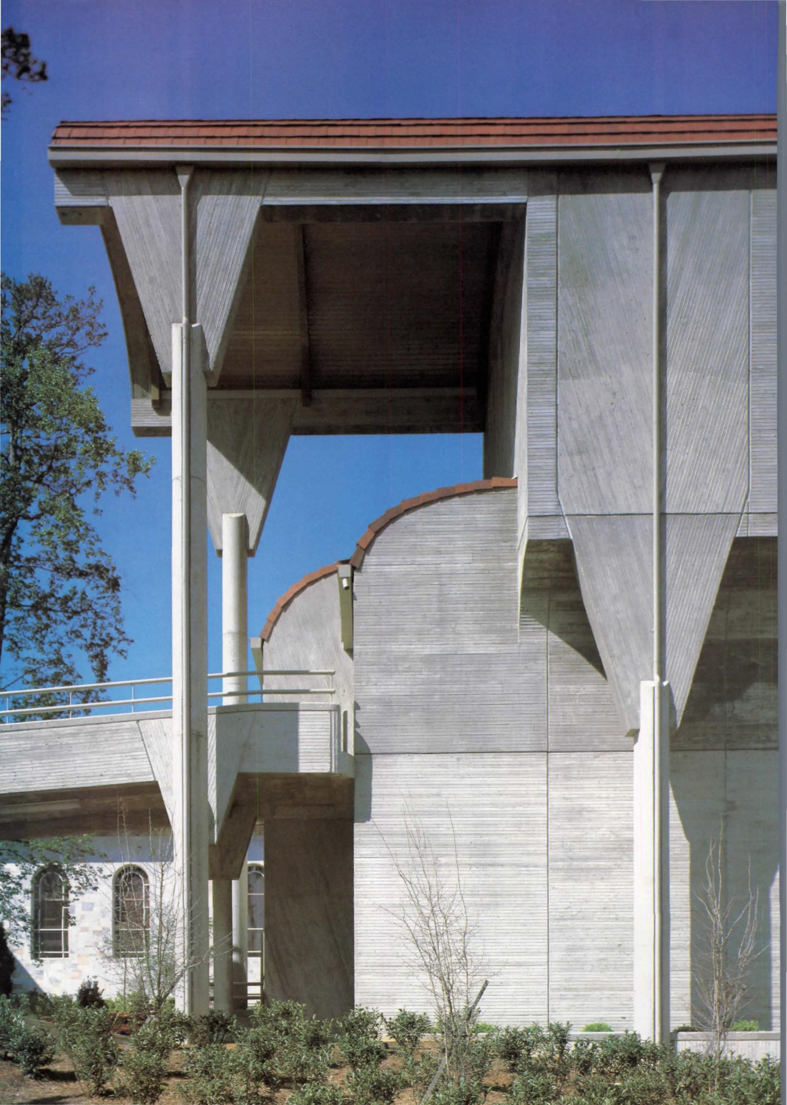
*The meticulously formed concrete (the contractor calls it "molded") used rough-sawn forms bordering on cabinetwork, and contrasts herringbone panels and haunches with a horizontal pattern. At the ends of vaults overlooking the courtyard (preceding page), the herringbones joyously emphasize*
