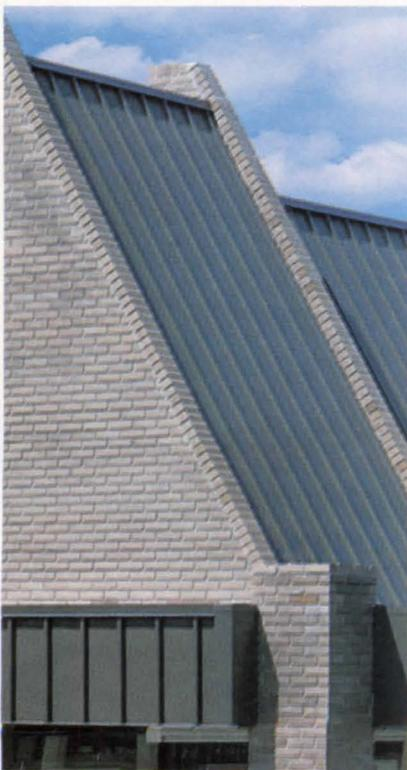
Howmet facing panels have a full 20 year, non prorated warranty . . . including labor. The baked on finishes are Desoto's Fluoropon® full strength Kynar 500®, with Koropon® Acid Rain Primer factory applied to aluminum or steel. It is guaranteed against chalk and fade regardless of the roof pitch from 0° to 90°. The finishes will not crack, check, peel or lose adhesion.
