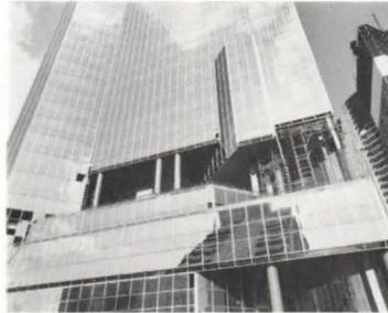
There are only 16 typical winged floors in the 35 stories of Tower 1. The four plans show how the tripod columns are incorporated into the building, and how, at the seventh level, the inboard column of the tripod has been omitted, leaving clustered pairs. The columns are 10 ft apart and 35 ft from the next pair. Notches at levels six and seven admit daylight to a skylight over the bank's atrium.
