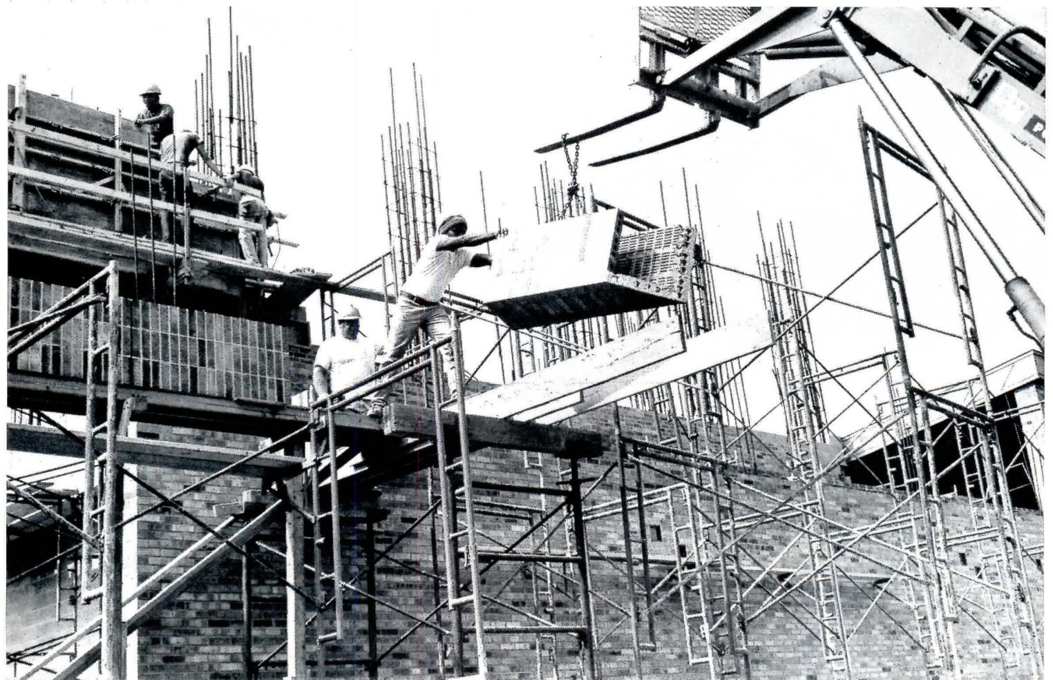
above them. Typical reinforcing for these beams is two no. 6 bars top and bottom. (Bond beam reinforcing is one no. 4 bar top and bottom.)
