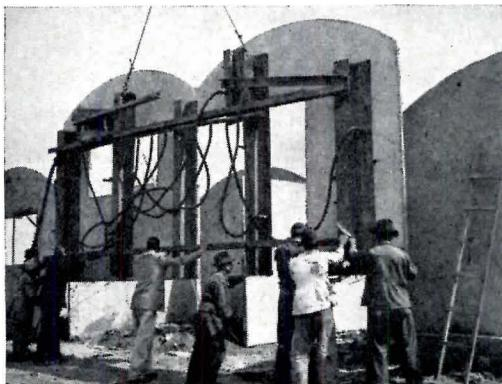
Vacuum equipment "pre-dries" each layer of concrete before the next is poured (photo far left). Later the same equipment is attached to a crane and used to hoist the pre-cast elements into place.
