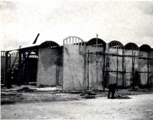
*Openings for doors and windows — and even glazed skylights as in the shell at right — are formed into the elements as they are cast. To eliminate tie rods and speed erection, column capitals and upper wall sections follow the curvature of the shells they support.*
