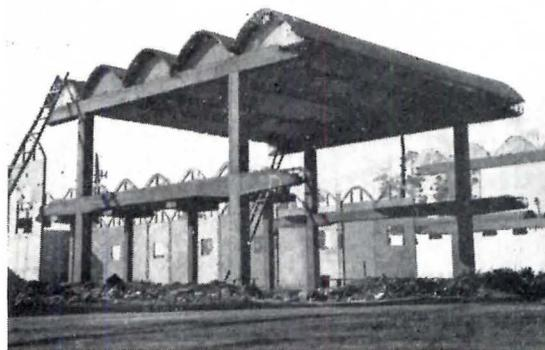
bay spacing need not exceed the combined width of two barrel shells, the columns are formed with radiating arches which support a shell on each side of the column; if more than two shells are needed to roof a bay, adjacent columns are spanned by a beam which is “scalloped” with arch sections that support as many shells as are required.
