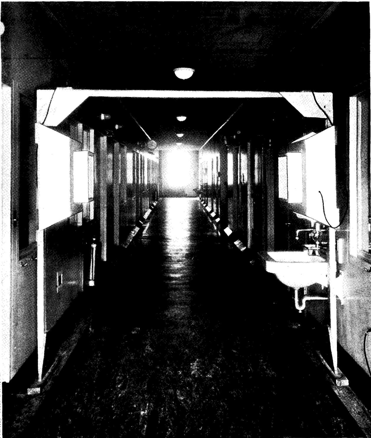
A barrier of ultraviolet light across the corridor of the isolation unit of the Children's Hospital in Boston, Massachusetts. Tests have shown that such screens can be made practically impervious to air-borne bacteria.
