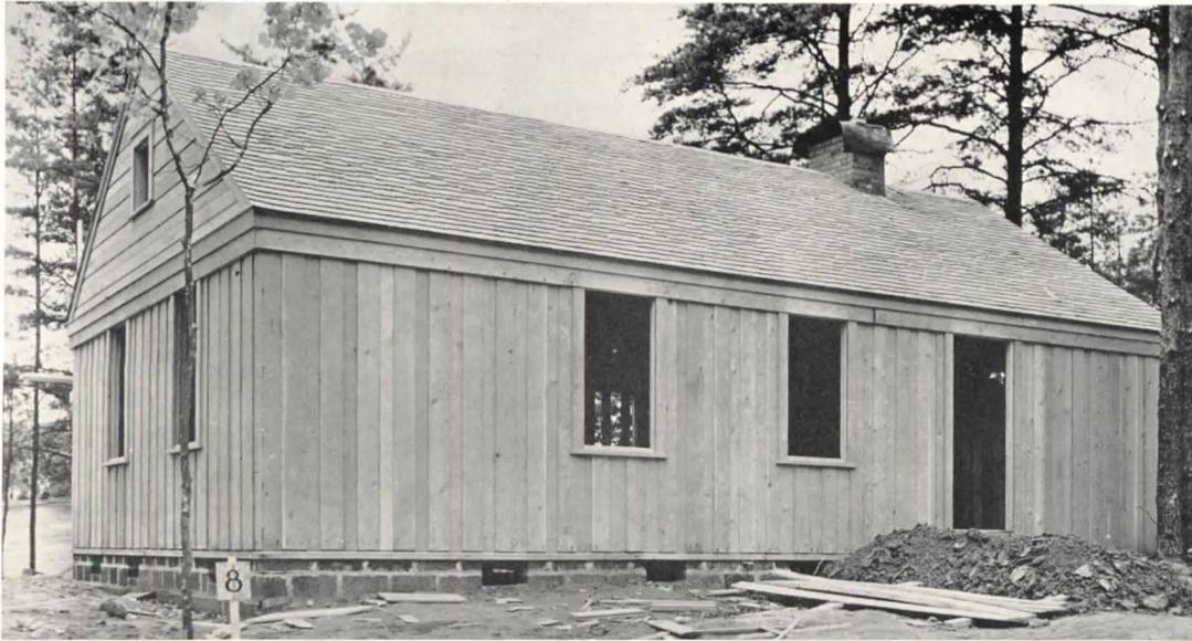
House built according to the Palisade system, which uses nominal 2-in. planking to form walls and subfloors. Planks in typical wall and in one type of floor are tongued-and-grooved, and staggered; double-faced plywood partitions approximately 2 in. thick have also been developed. Additional information is given on page 89.
