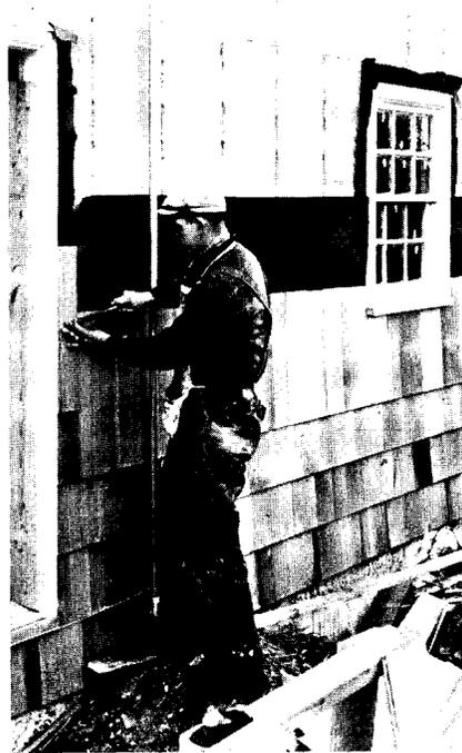
Shingling the Edward house. Use of plywood and prevention of wind-leakage at openings reduced air-infiltration so greatly that use of wall insulation was considered uneconomical. However, roof insulation was included. Specifications were prepared in cooperation with the Oregon-Washington Plywood Co., using the "Uniwall" system.
