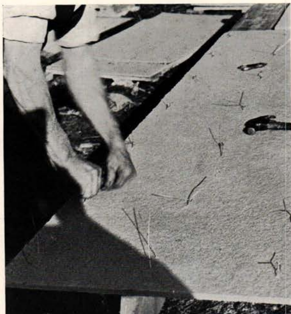
FIGURES 3 AND 4 (BELOW) — BONDING WIRES ARE APPLIED TO CELOTEX (THEN PLACED IN THE FORMS) SO THAT CONCRETE WILL HOLD THE INSULATION PERMANENTLY IN PLACE.
