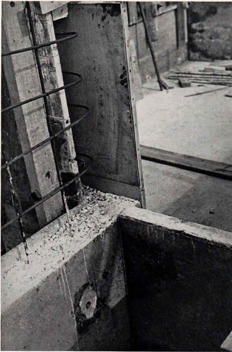
FIGURE 5 — DETAIL OF WALL REINFORCING SHOWING HOW EXTERNAL FORMWORK AND FIBER-BOARD LINING ARE POSITIONED.
