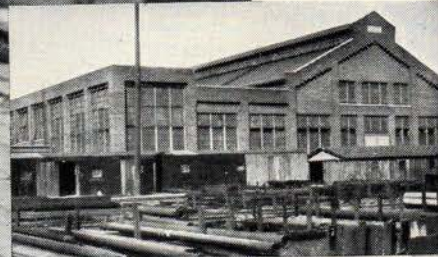
J-M Smooth Sur- faced Asbestos Roof on the Beech Grove, Ind., Shops of the Big Four Railroad. Applied 1910. Photo- graphed 1935. Still in excellent condition.
