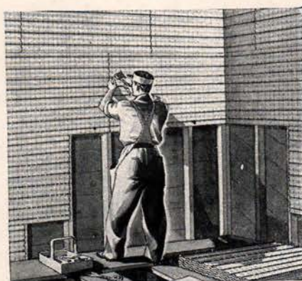
Reynolds Ecod Fabric is supplied in sheets. Quickly installed Metallated Ecod combines efficient insulation with metal plaster base for only 6/10 of a cent extra per square foot, over plain lath.
