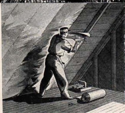
You apply Reynolds Metallation right over the rafters, roof joists, studs or sheathing. It is clean and easy to handle and install. Only snips, nails and a hammer are required.
