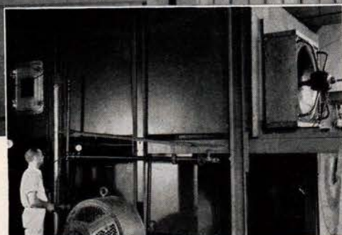
The giant air tunnel used for testing units. The new Venturafin Units deliver 10 to 64% more heat, 4 to 45% more air (depending on size of unit) with no increase in horsepower.
