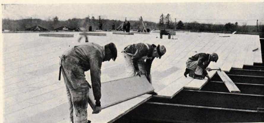
Erecting PLANK roof on the Artillery Transportation Storage Shed, the Armory Commission, Commonwealth of Massachusetts. J. Theodore Whitney, Engineer.
