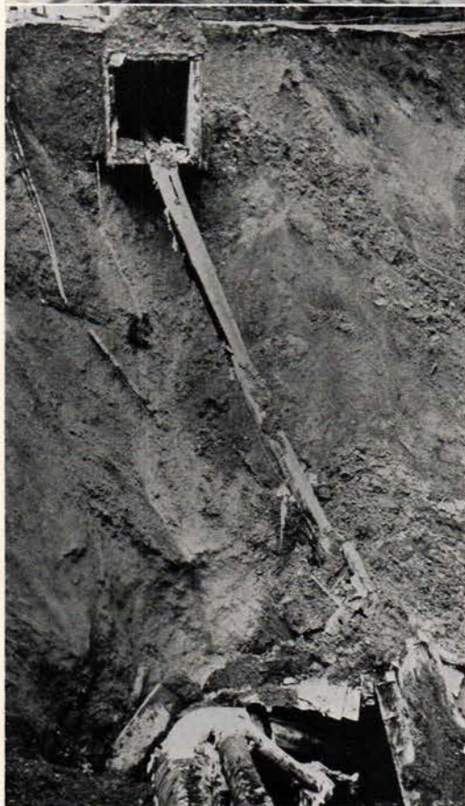
Above: A view looking across the gap from one broken end of the tunnel to the other. Below: A photo which gives a clearer idea of what happened to the tunnel and pipe lines.
