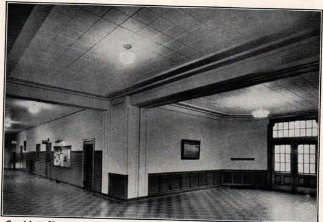
Corridor of Irvington School, Portland, Ore. Acousti-Celotex Sound Absorbing Tiles on the ceiling subdue noise in these hallways where much of it originates. George H. Jones, Architect, Portland, Ore.
