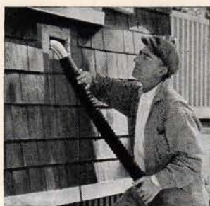
Applied to existing construction pneumatically
