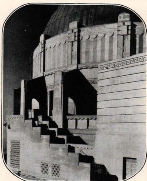
Detail of Griffith Observatory. Domes over the Planetarium and the Foucault Pendulum are of concrete and copper.
