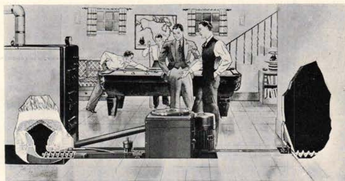
Iron Fireman automatic anthracite burner feeds coal from bin to fire, removes ashes
