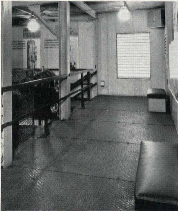
In the elevator house—display room of the Otis Elevator Company—floors, stairs, and landings are of Inland 4-Way Floor Plate.
