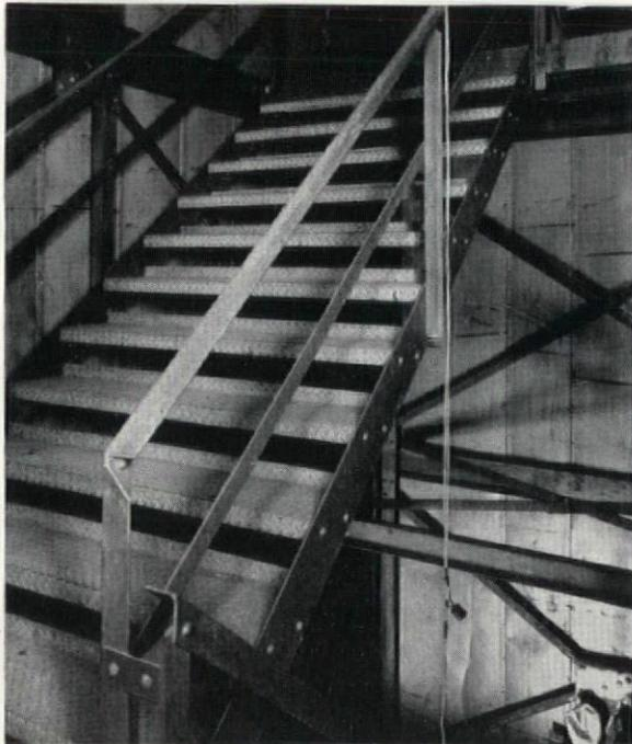
The emergency stairway from the ride level (220 feet) to the ground is of Inland 4-Way Floor Plate.
