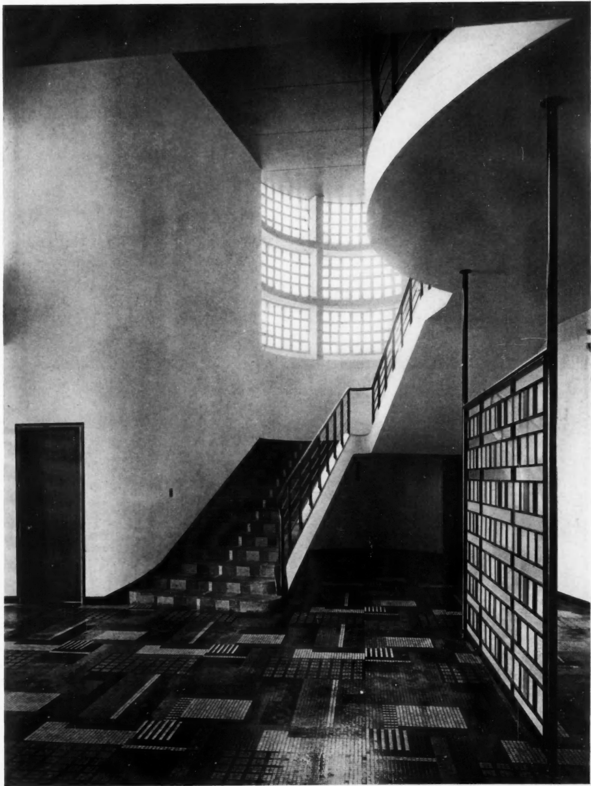
Main Stairway. Mosaic tile floor and tile base.
