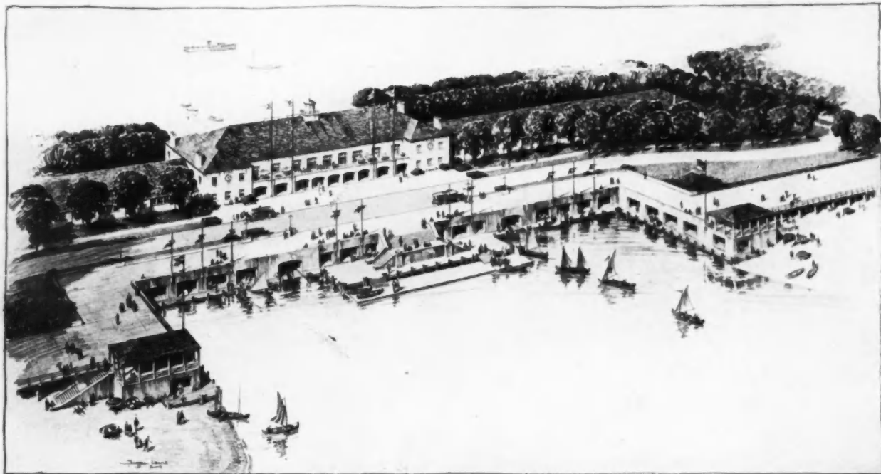
Bird's-eye view of the Inlet Yacht Club showing Yacht Harbor beyond. Floats for launching sailing canoes are shown in front. At each side is a double-deck boardwalk. Beach storage for 500 canoes is provided.
