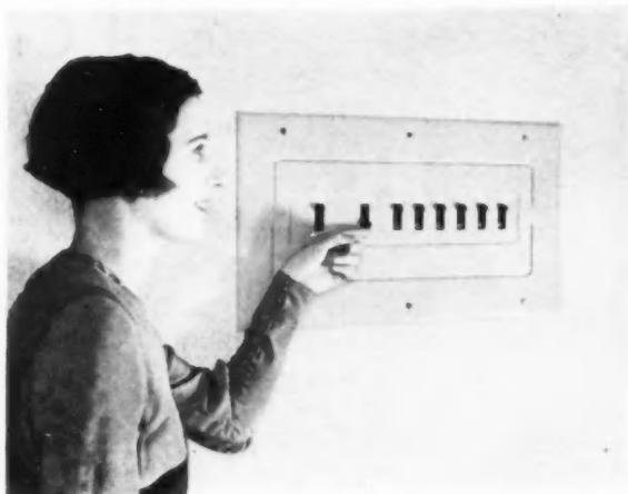
No-Fuse Load Center located in an accessible place in the house.
