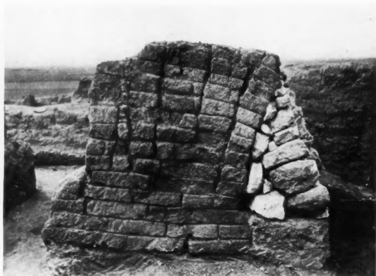
A TYPICAL BUILDING (LEFT) AND A SECTION (RIGHT) OF TRUE ARCH CONSTRUCTION OF MUD BRICK FOUND ON EIGHTH LEVEL OF TEPE GAWRA, IRAQ.
