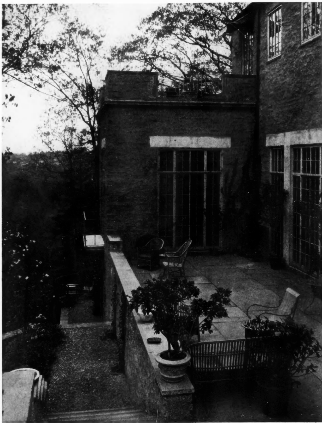
Terraces and outside steps are of flagstone.
