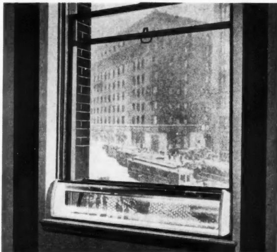
"Silentaire" sound excluder for double-hung windows. Truscon Steel Company.
