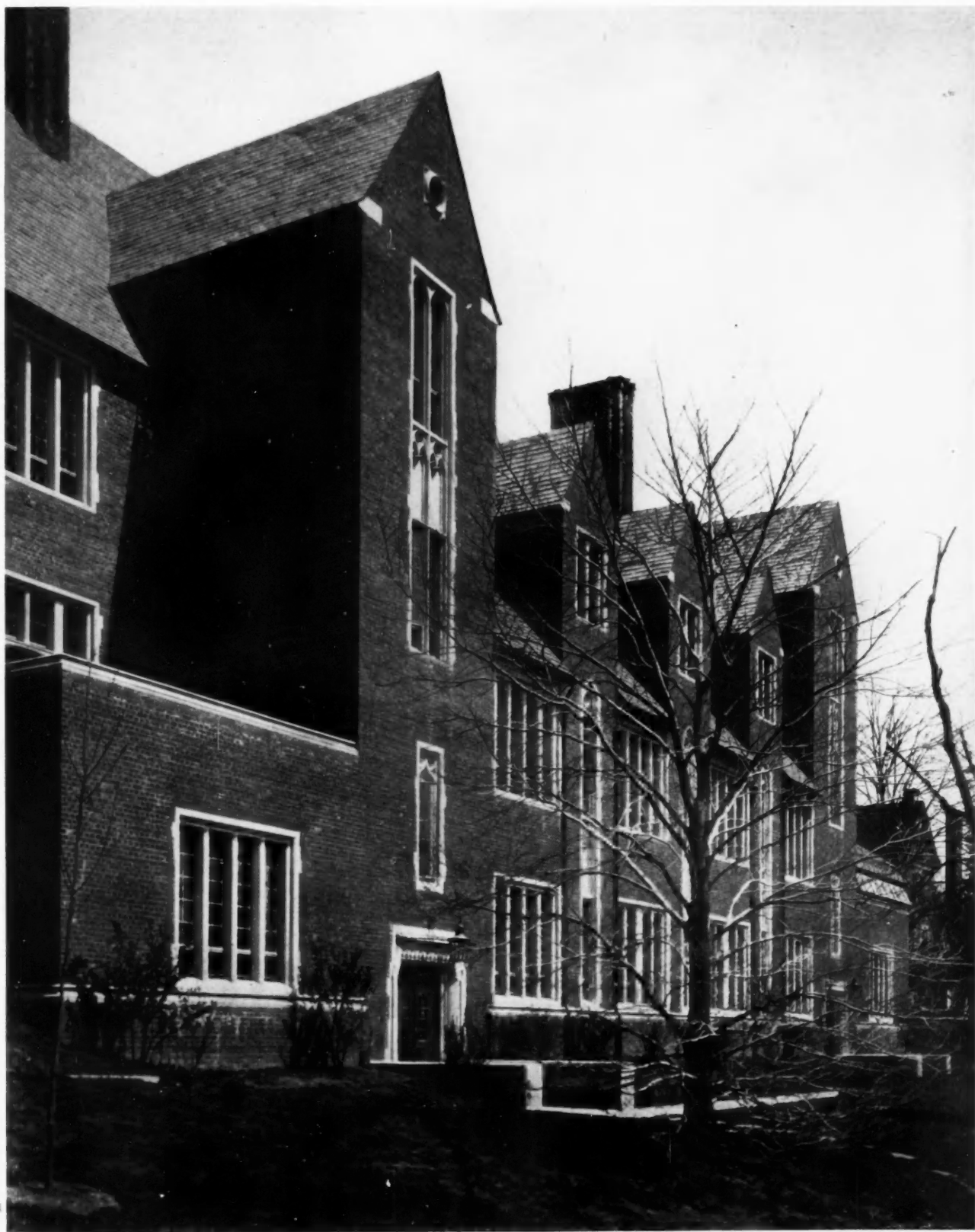
HARRY ELKINS WIDENER SCIENCE BUILDING THE HILL SCHOOL IN POTTSTOWN, PA. CHARLES Z. KLAUDER, ARCHITECT
