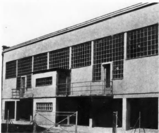
FIG. 8 LUXFER CONCRETE FRAME WINDOWS. TRANSFORMER STATION, PFALZ.
