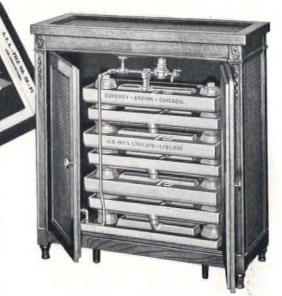
\$150 to \$225, f. o. b. factory, installation extra, in beautiful metal cabinet. Supplied also for recessing in wall. Types and sizes for any building heated by steam, hot water, or vapor. Water fed in at the top spreads out over horizontal first section, the overflow going down and spreading out over the second section, and so on until the last section is reached.
