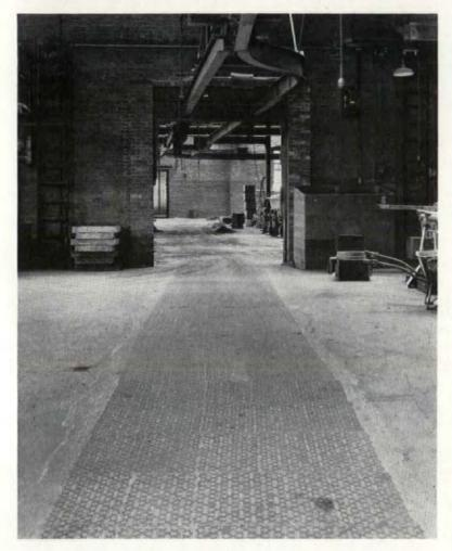
Above is pictured a section of the foundry gangway at a prominent Rhode Island plant. The gangway consists of approximately 5,500 sq. ft. of Snead No. 30 Heavy Duty Armor Grids and has been installed for about two years. A careful inspection recently made revealed the surface to be in really excellent condition despite the terribly heavy traffic to which it has been subjected. We make the prediction that this gangway will be as satisfying 20 years after installation as it is right now.
