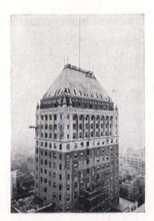
Tower portion of Newark & Essex Bank Building. Alberene Stone Spandreis used at 32nd and 33rd floor levels—on all four elevations.
