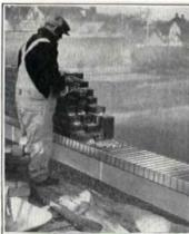
Rebuilding Parapet with Chen Flashing installed above the roof line
