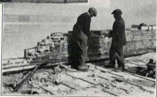
Top View—The Building Showing Parapet Partially Removed Lower View—Tearing down the leaky Parapet
