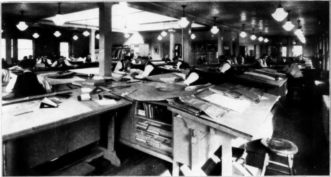
A corner of The Kinnear Manufacturing Company's Engineering Department
