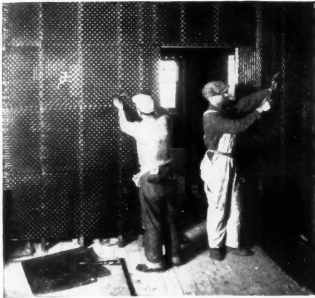
Arch Lath permits easy, quick application because of great rigidity
