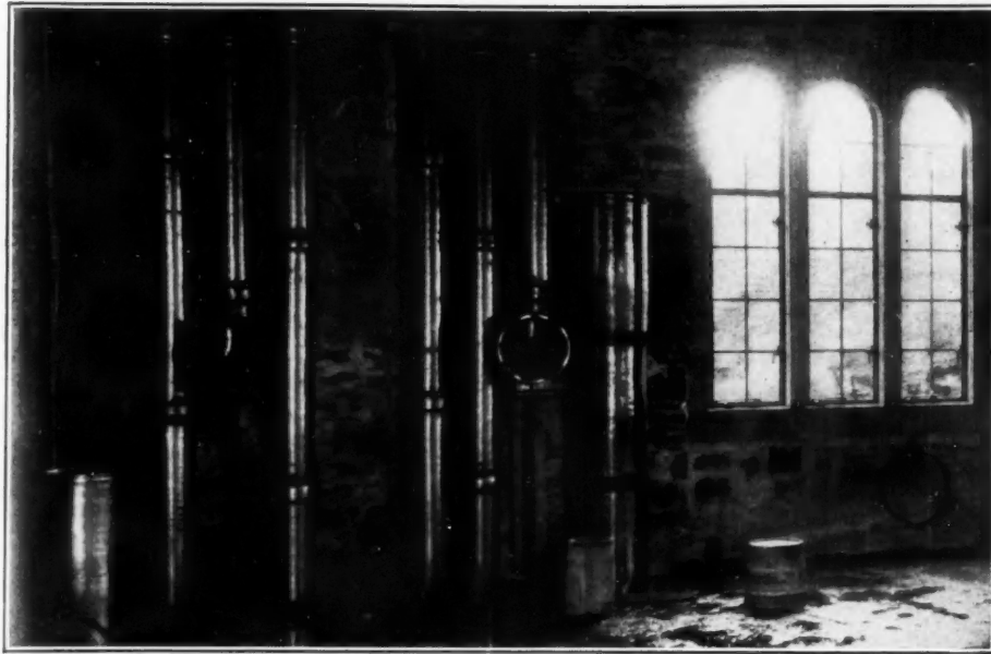
Knight-Ware 9-in. and 22-in. Bore Ventilating Ducts with Base Ells at Princeton
