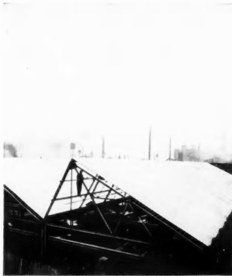
Mahon Steel Roof Deck installed on a new building for the Bohn Aluminum and Brass Corporation, Detroit, Mich.
