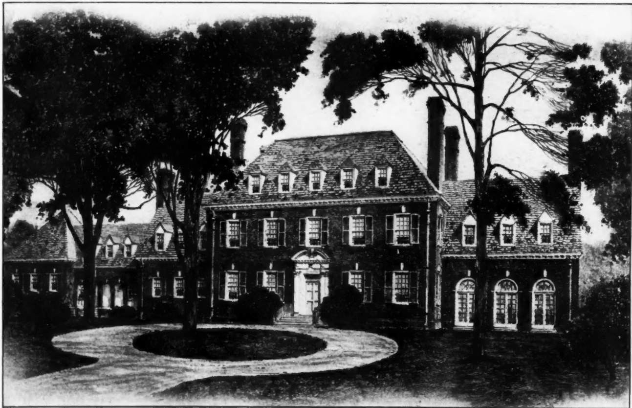
The home of Mr. H. W. Ellerson, Richmond, Virginia, insulated with Armstrong's Corkboard. W. Duncan Lee, the architect, says after the first winter, "Insulation has been thoroughly satisfactory . . . will pay for itself many times."
