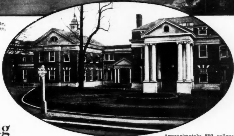
Approximately 800 gallons of Barreled Sunlight were used by the University of Virginia for interior painting in the Hospital Group of Buildings and the new Medical School
