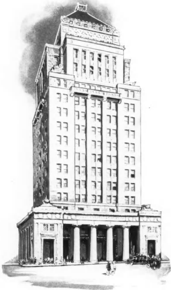
Cincinnati Gas & Electric Company Cincinnati, Ohio
