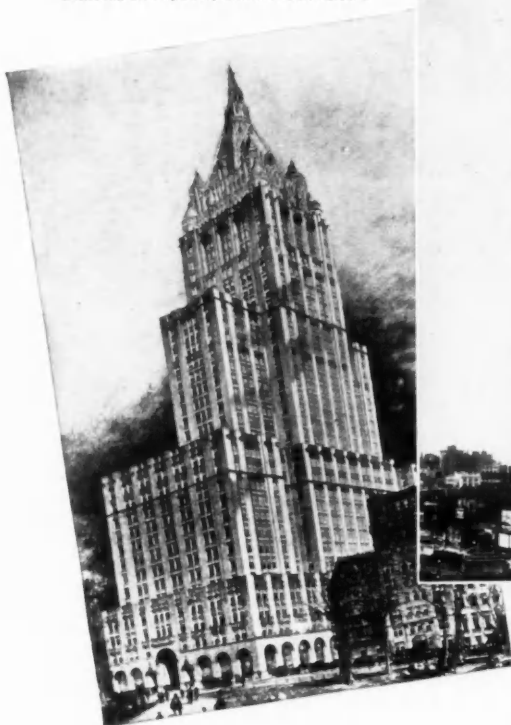
New York Life Insurance Building New York, N. Y. Cass Gilbert, Architect Starrett Bros., Inc., General Contractors
