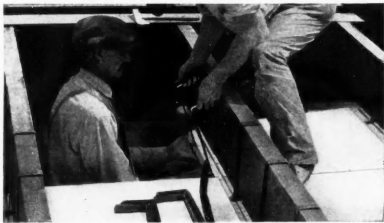
Suspending Ceiling Slabs by hangers from steel floor members, which may be rolled shapes or open-web welded joists.
