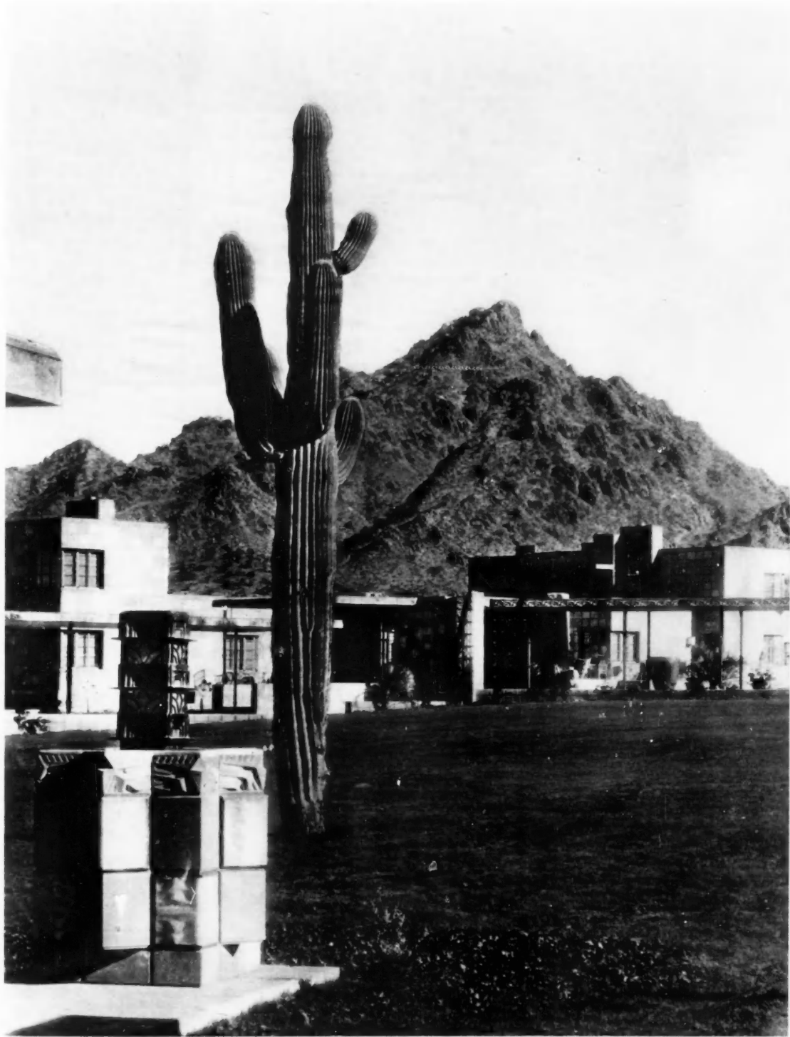
VIEW OF BUNGALOW FROM PATIO
