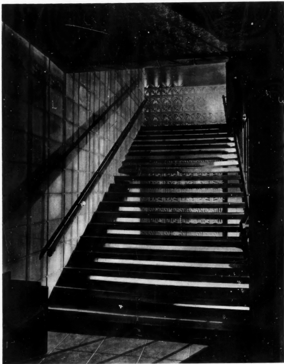
STAIRWAY TO BASEMENT Arizona-Biltmore Hotel, Phoenix, Arizona ALBERT CHASE MCARTHUR, ARCHITECT
