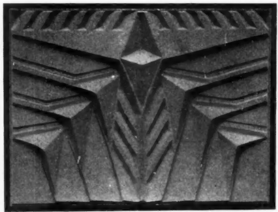
SINGLE BLOCK UNIT IN CAST CONCRETE
