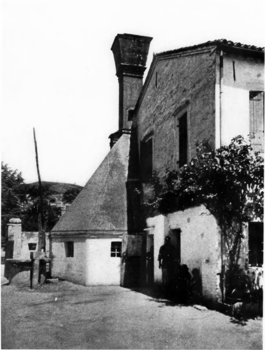
FIG. 6. VENETIAN KITCHEN CHIMNEY AT MIRANO
