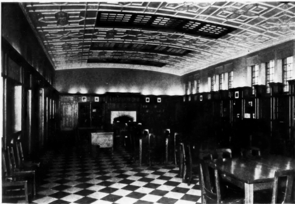
Library J JEFFERSON INTERMEDIATE SCHOOL, DETROIT, MICHIGAN Malcomson & Higgenbotham, Architects
