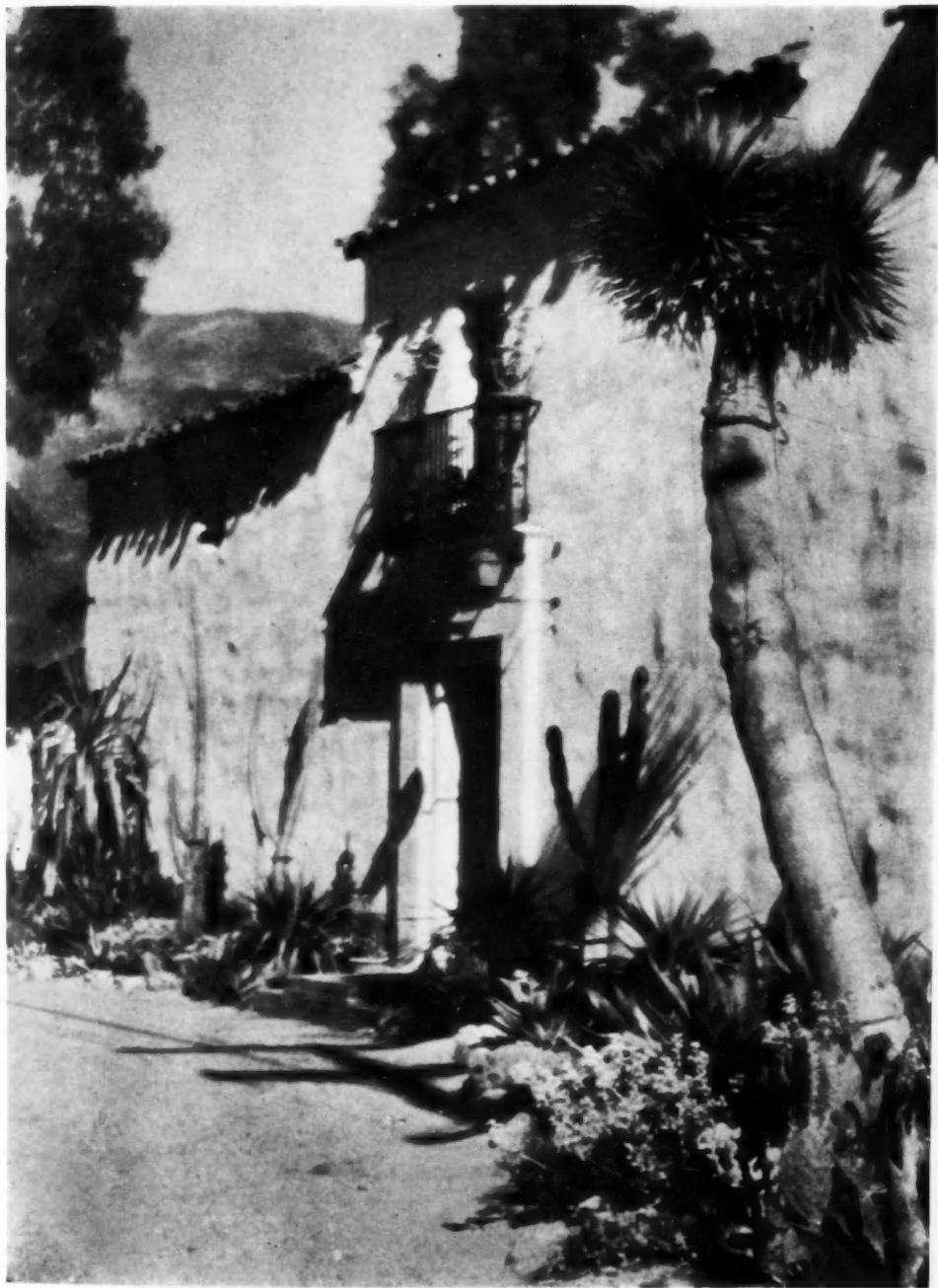
RESIDENCE OF CRAIG HEBERTON, ESQ., MONTECITO, CALIFORNIA George Washington Smith, Architect
