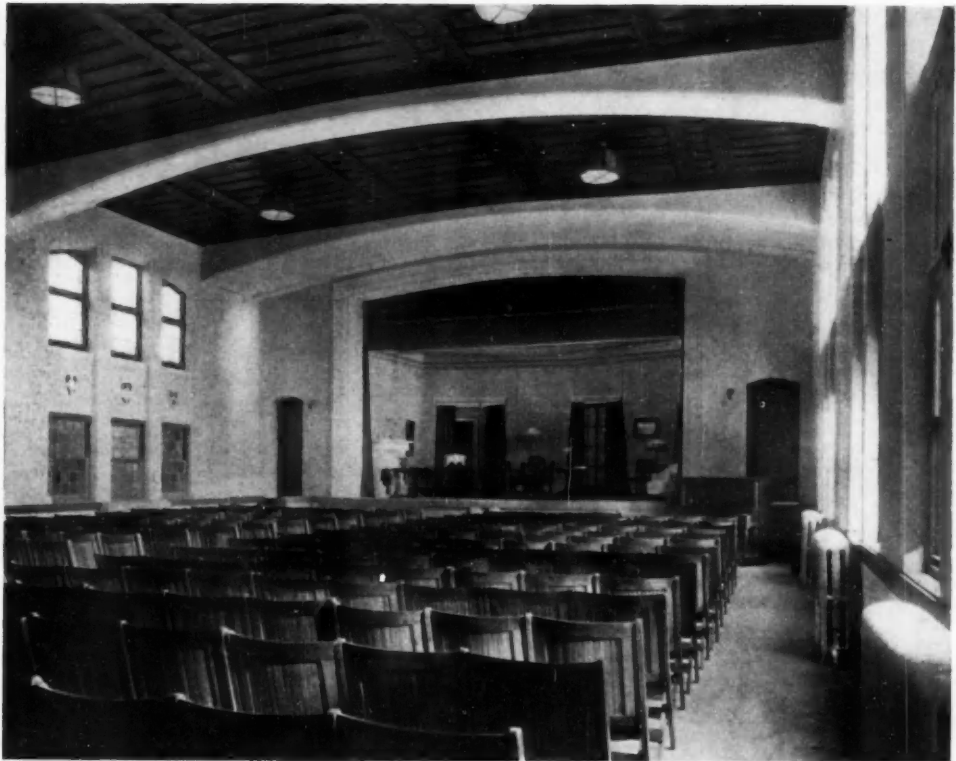
Social Hall ST. LUKE'S PARISH HOUSE, EVANSTON, ILLINOIS Tallmadge & Watson, Architects
