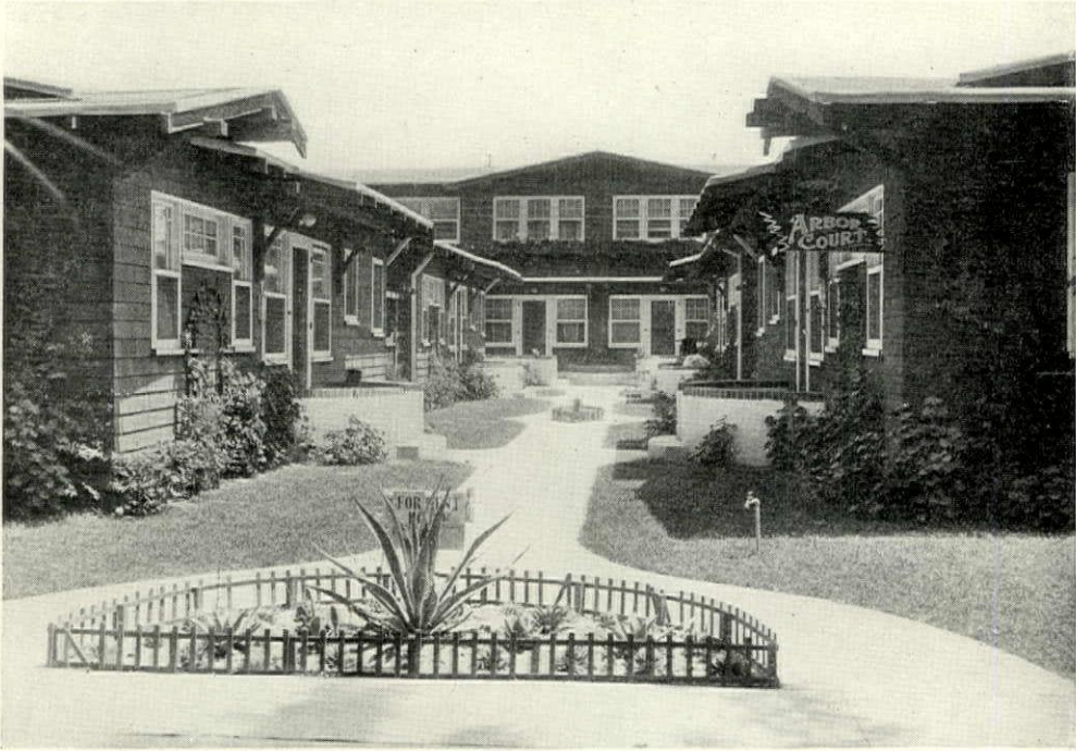
FIG. 5. FOUR SINGLE HOUSES AND ONE TWO-STORY DOUBLE HOUSE ON A PLOT 60 BY 140 FEET.
