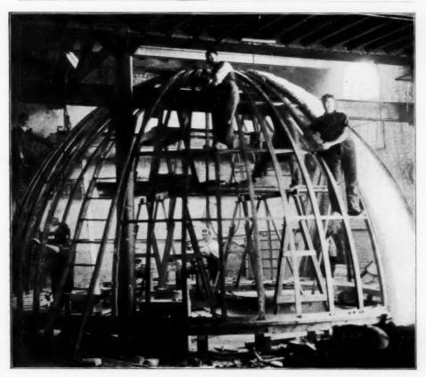
TOTAL HEIGHT 24 FT. 0 IN., DIAMETER 22 FT 0 IN. COLOSSAL CAST BRONZE DOME FOR MAUSOLEUM
