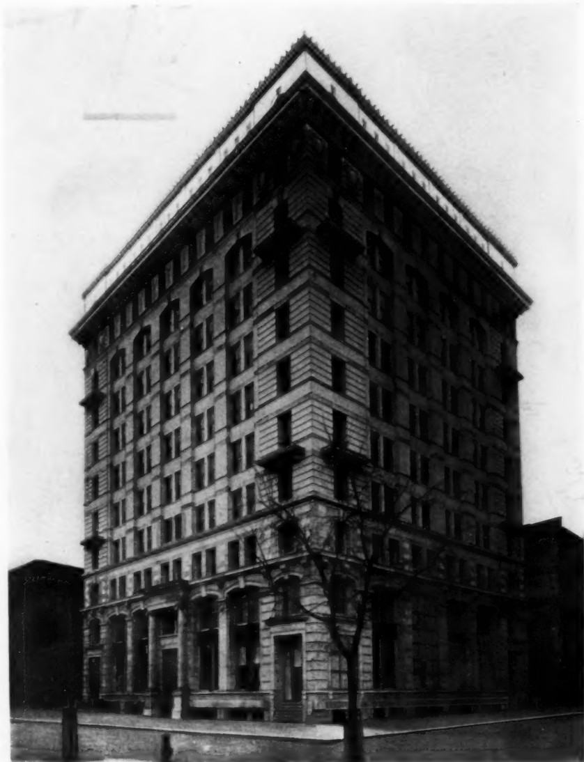
THE BATTERY BUILDING.
