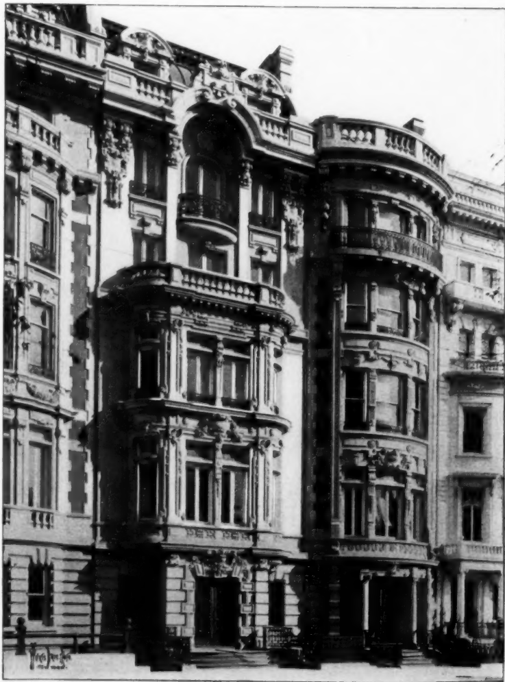
NOS. 1007 AND 1008 FIFTH AVENUE. New York City.
