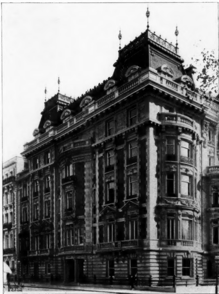
NO. 1009 FIFTH AVENUE. (The Duke Residence.)
