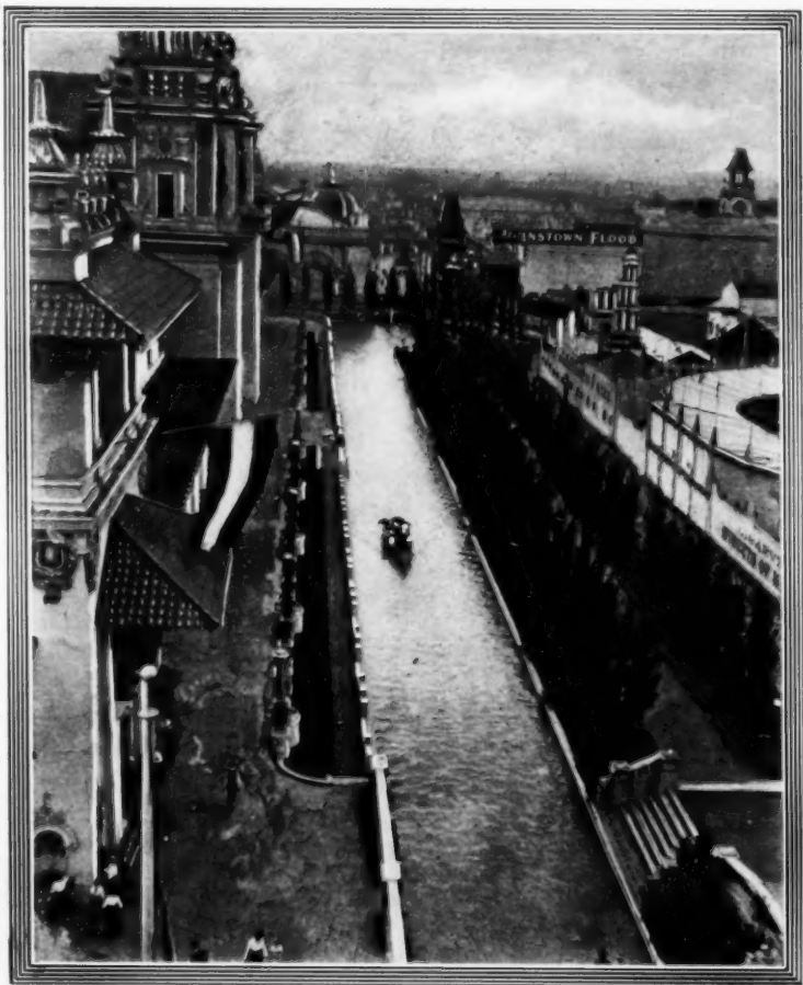
THE CANAL FROM THE ELECTRIC TOWER.
