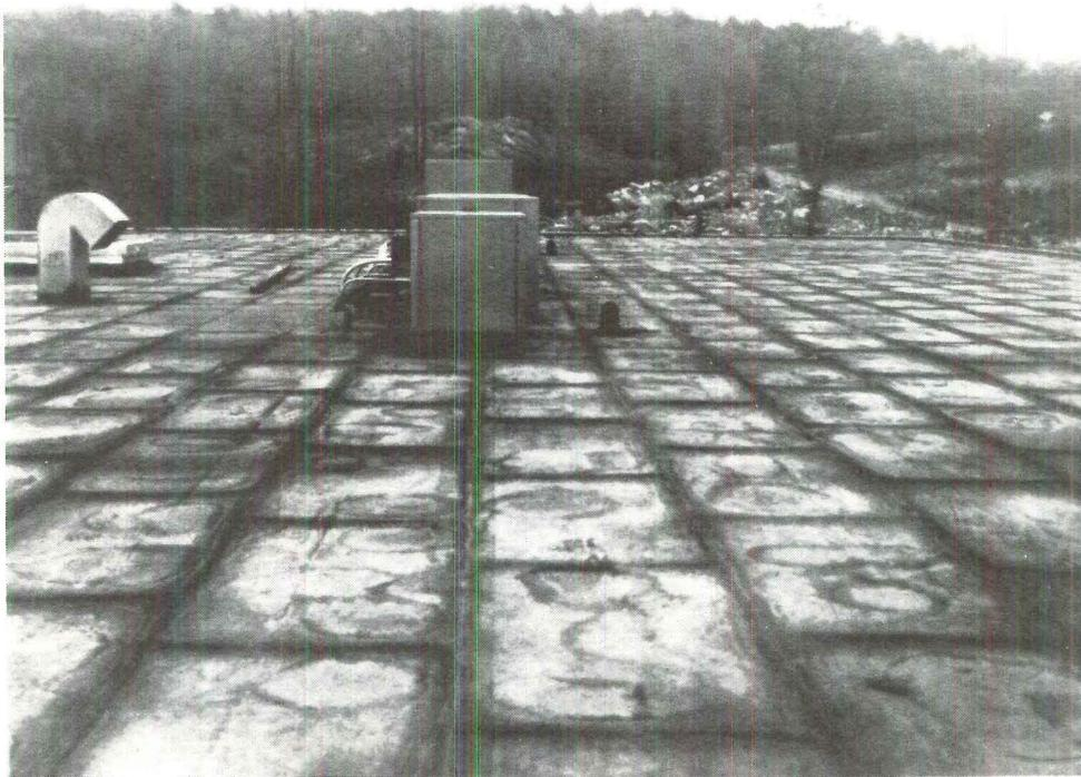
Insulation joints are built-in failure points in roof systems.
