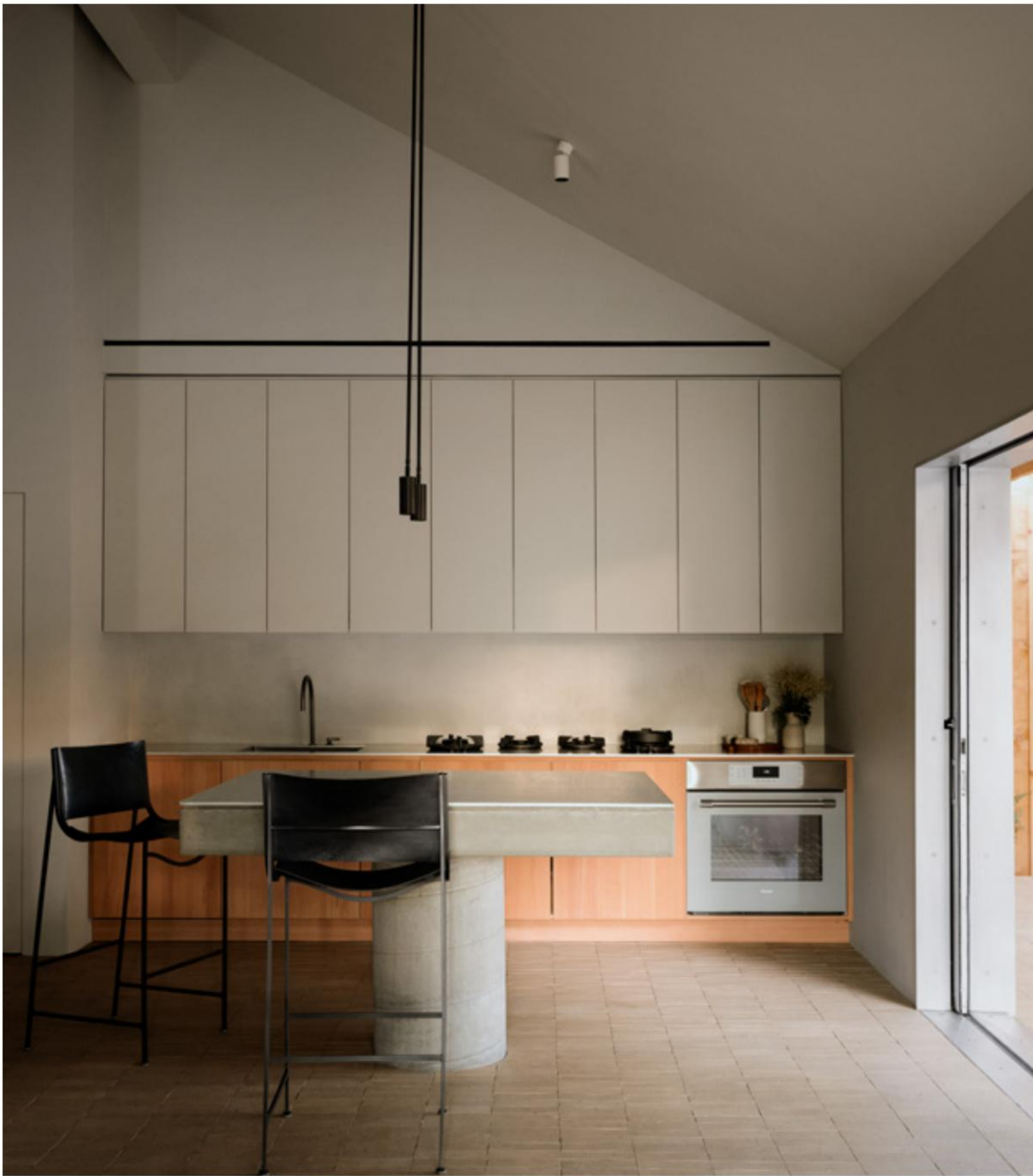
ABOVE The kitchen island is cast-in-place concrete and located adjacent to a slider that opens to the deck.
