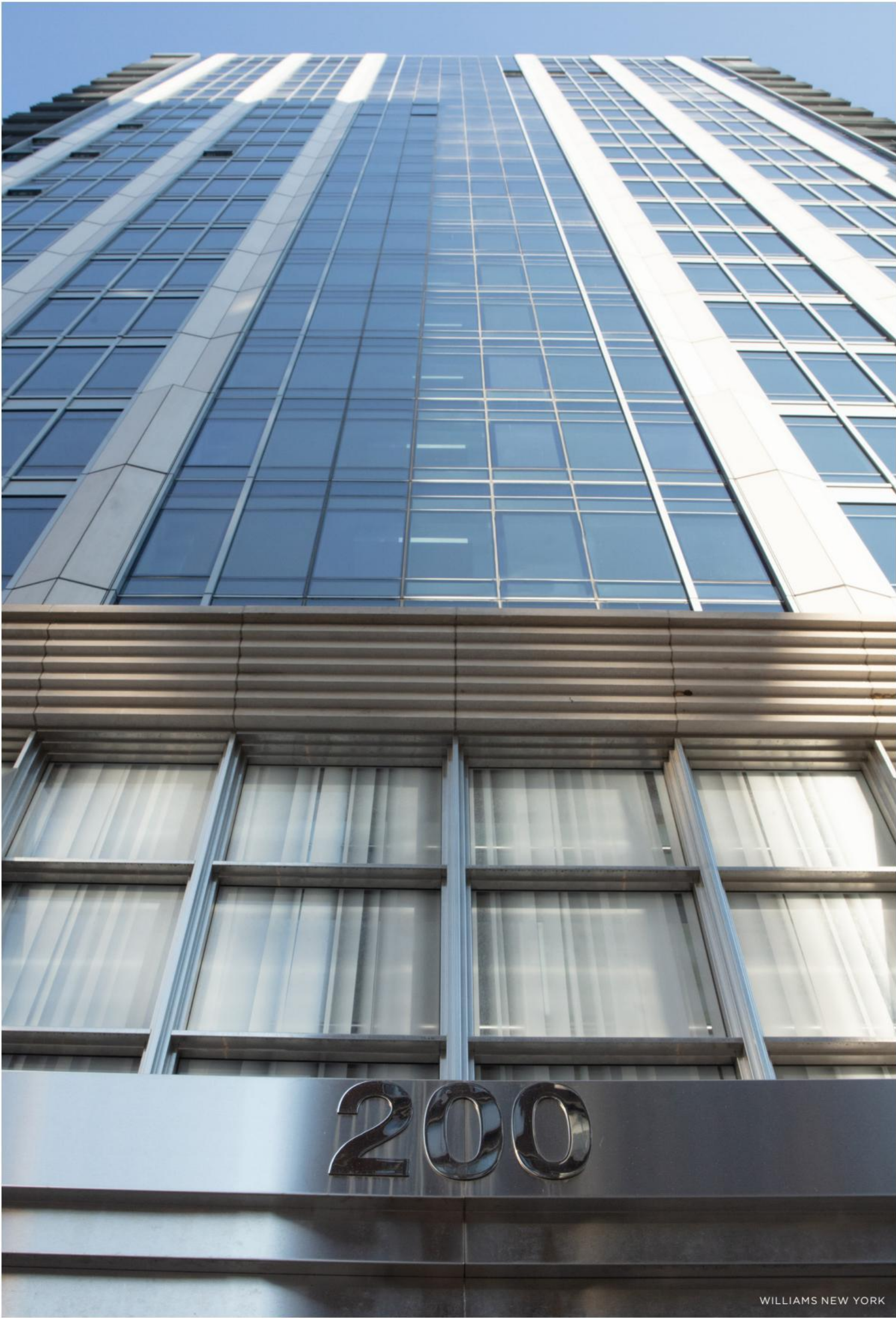
At Elkus Manfredi's 200 Amsterdam tower, a direct-to-glass design simulates interior draperies, creating privacy while allowing ample daylighting.
