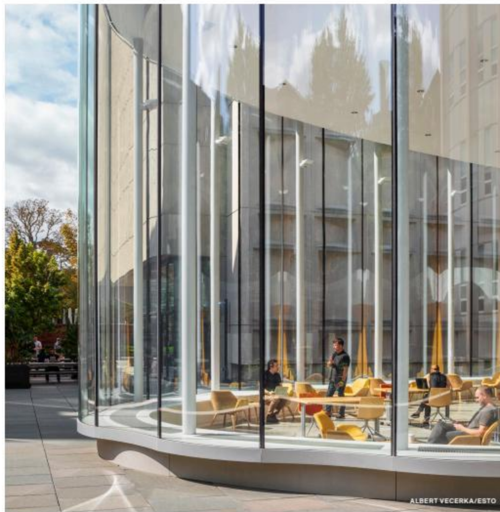
The Tsai CITY at Yale features 22-foot-tall mullionless structural glass panels.
