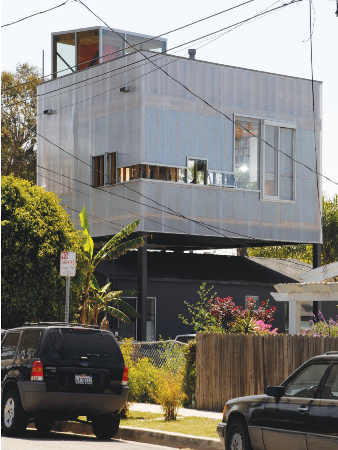
On a nondescript back street in Venice, a trapezoidal-shaped, polycarbonate-clad, second-story addition punctuates a row of single-story homes. Sitting on a "table" composed of five steel beams and seeming to have no connection to the original painted-gray, slanted-roof
