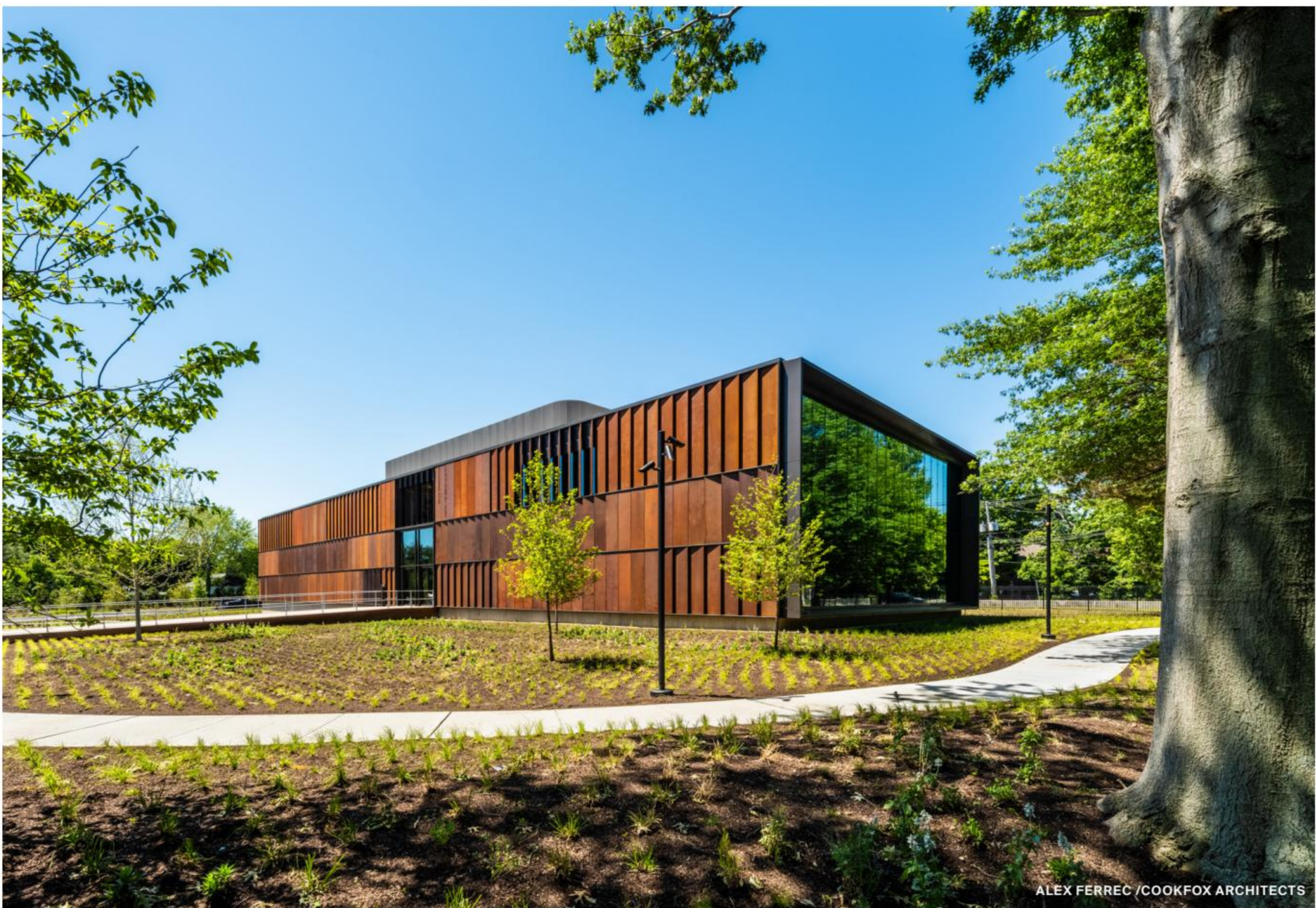
Facing page: The facade features weathering-steel rainscreen panels that reference New Jersey's industrial heritage, often cited in Springsteen's lyrics. Above: The building is located on Monmouth University's campus, in West Long Branch, New Jersey, close to places that informed Springsteen's early career.
