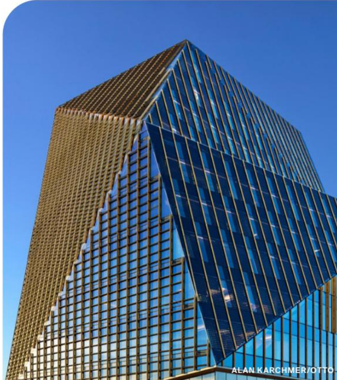
1 As seen in SmithGroup's Virginia Tech Academic Building One, photovoltaic glass also provides passive shading due to the solar cells embedded in the units.
