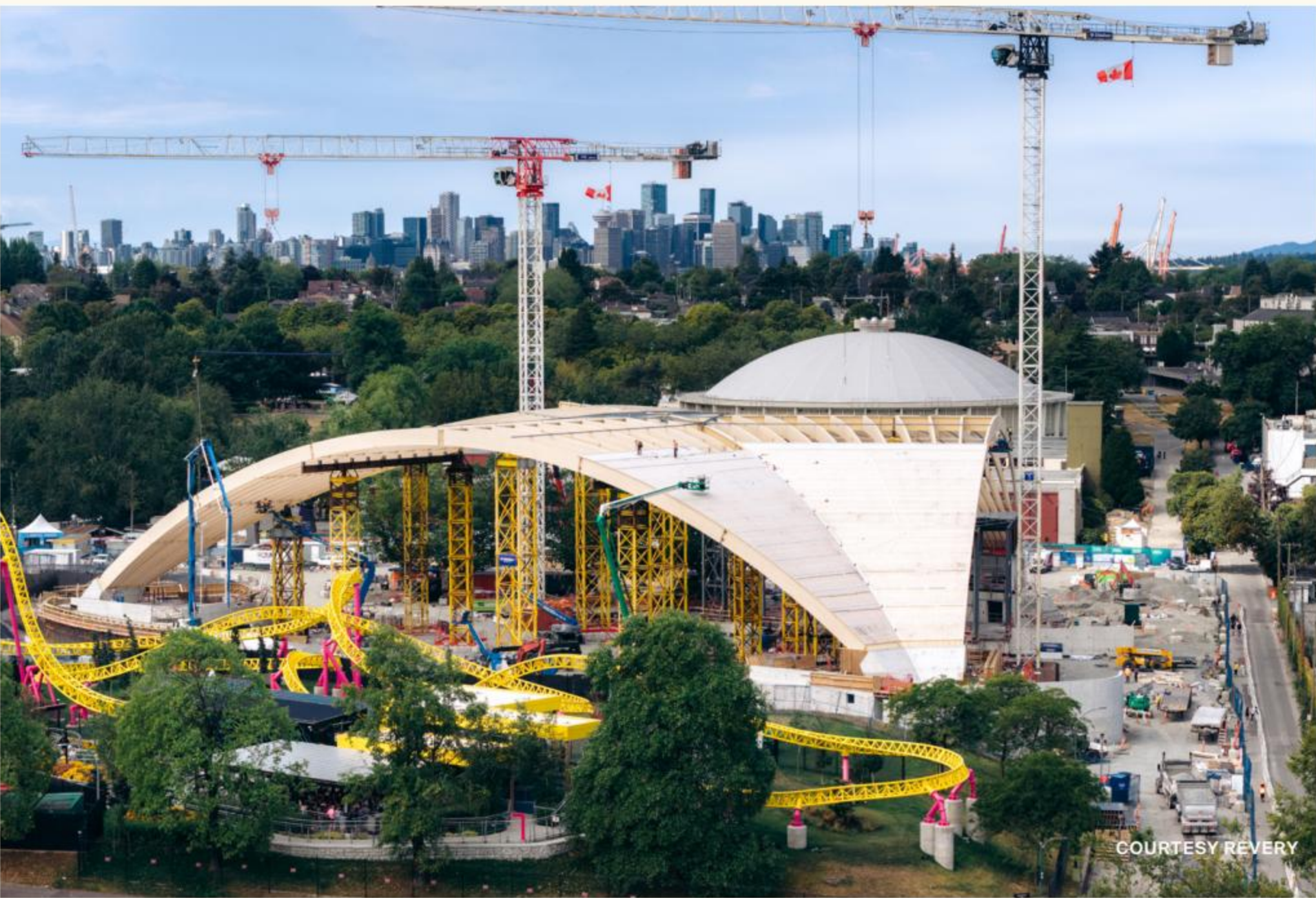
Revery Architecture's Freedom Mobile Arch covers the 10,000-seat venue with a 105-meter Douglas fir roof, arranged in a starburst pattern and landing on only three points.
