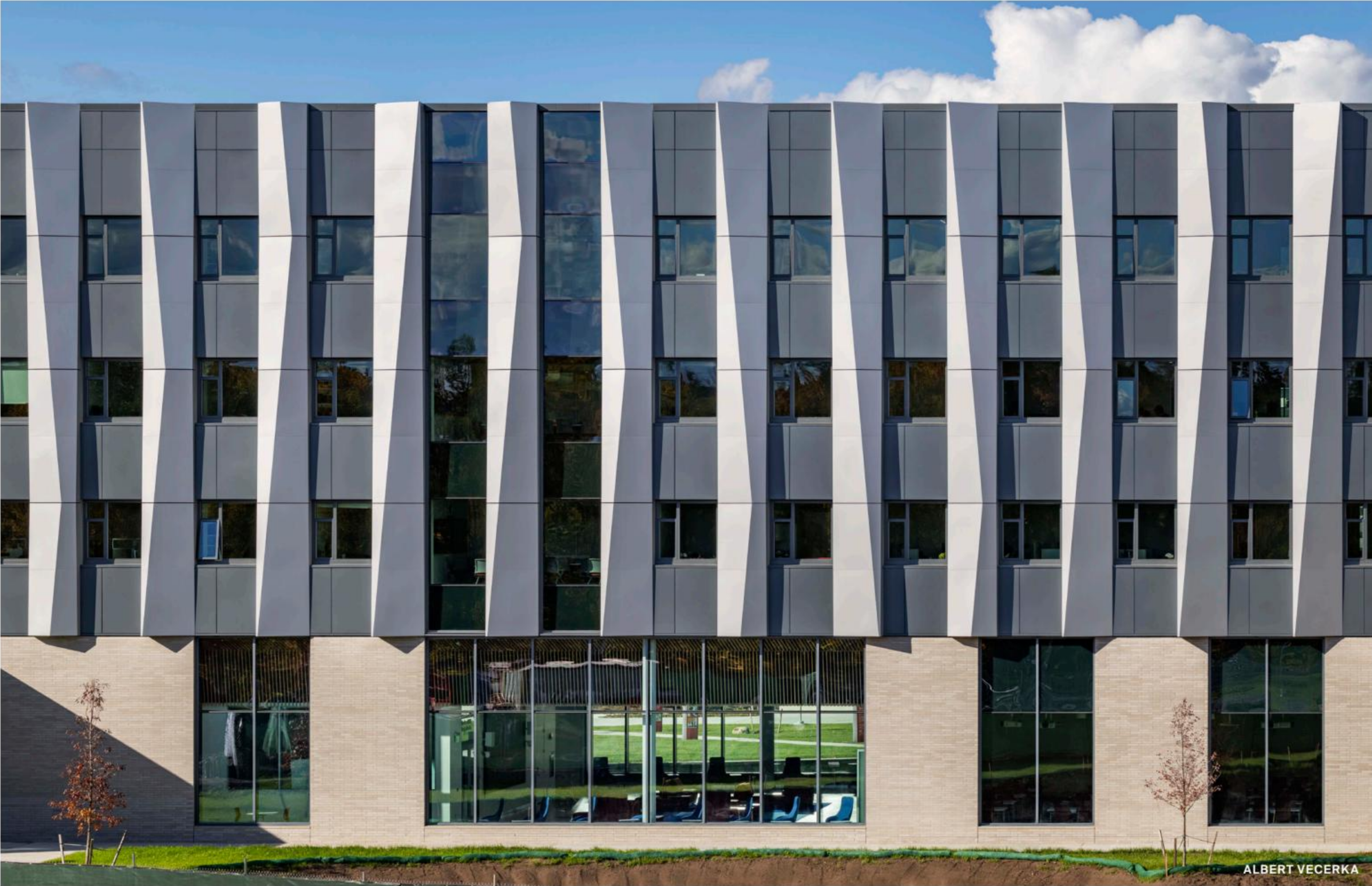
Left: Across the facade, punch windows are animated by sculptural metal fins in four configurations. Right: Inside, a heavy use of cross-laminated timber added much-desired warmth. Below: An underlying steel structure was used to achieve the undulating affect across the building facade fins.
