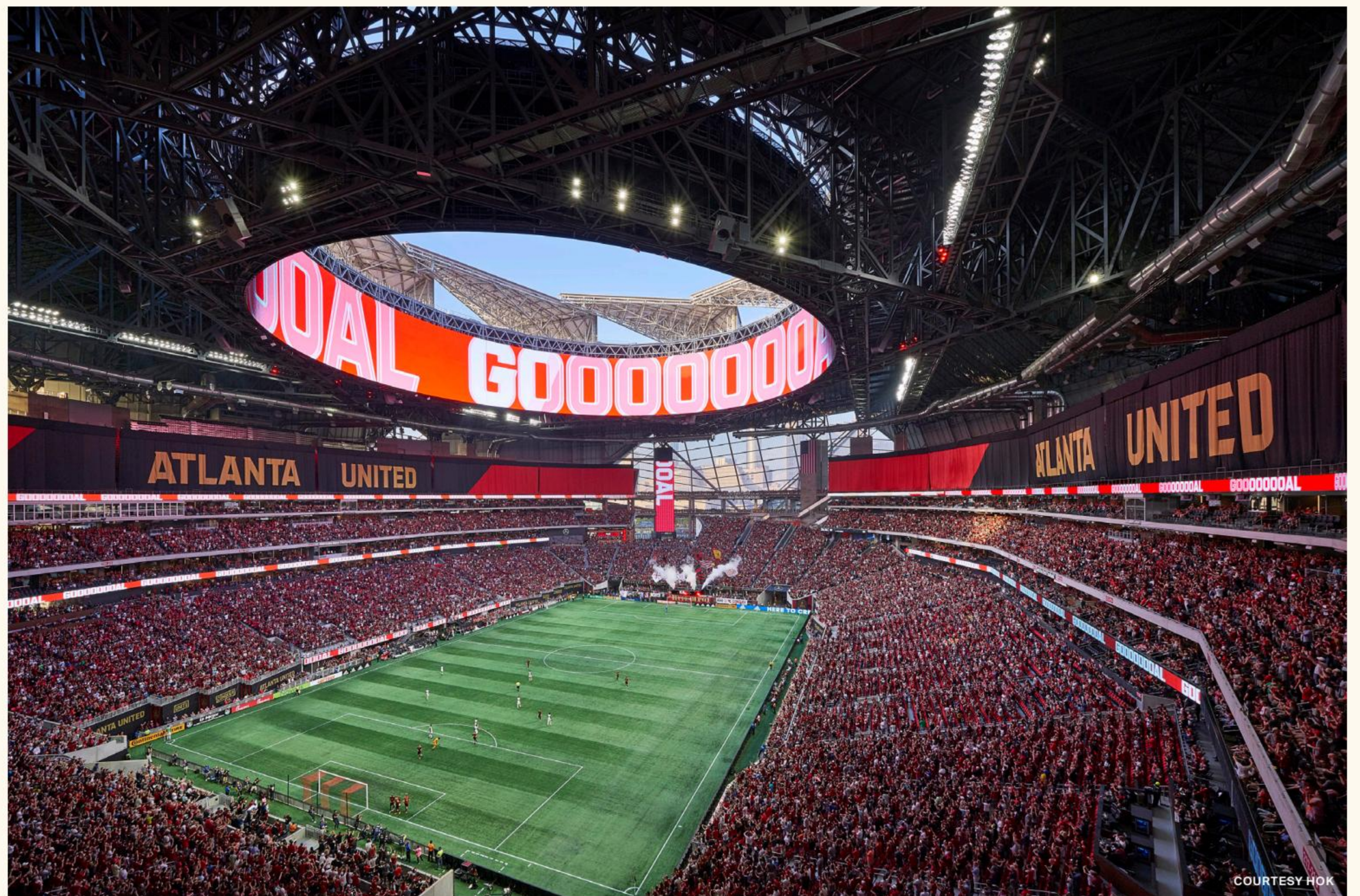
HOK's retractable roof opens like a camera aperture, with eight ETFE petals moving in unison along 16 tracks. The form was inspired by the Pantheon's oculus.
