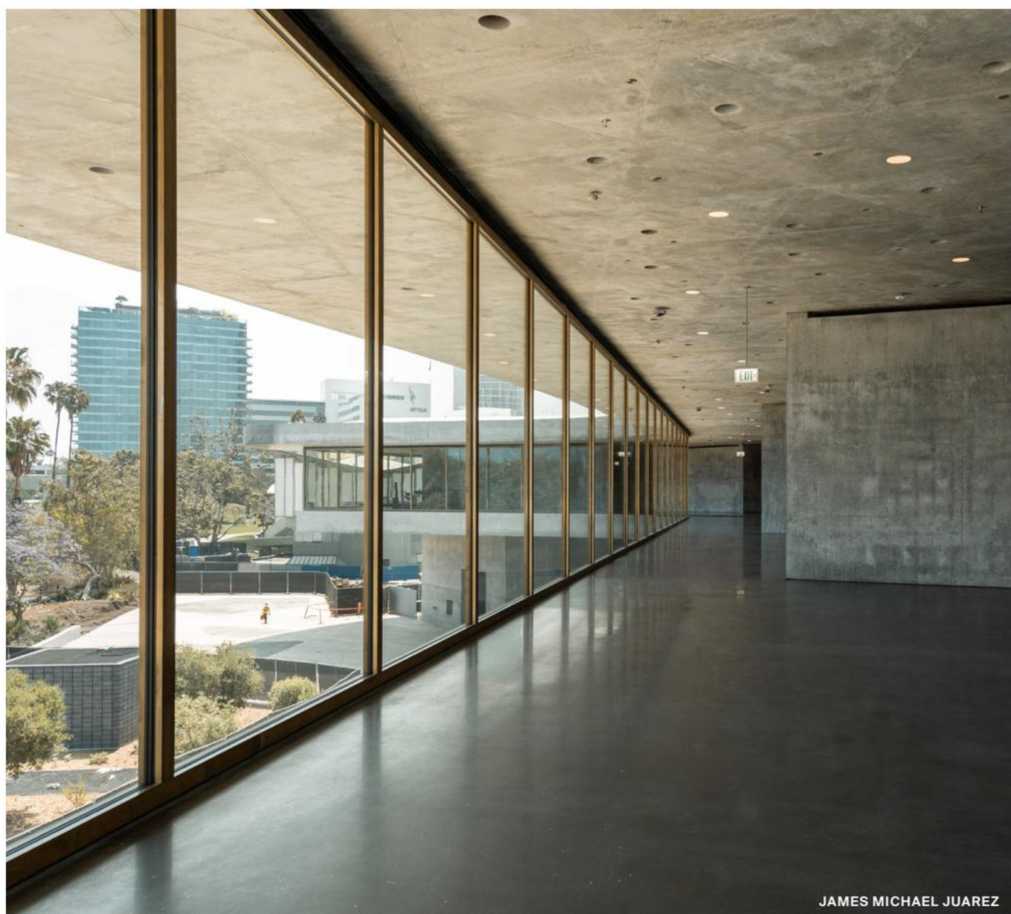
Left: The building's brass window wall, made by seele, wraps the entire facade.
