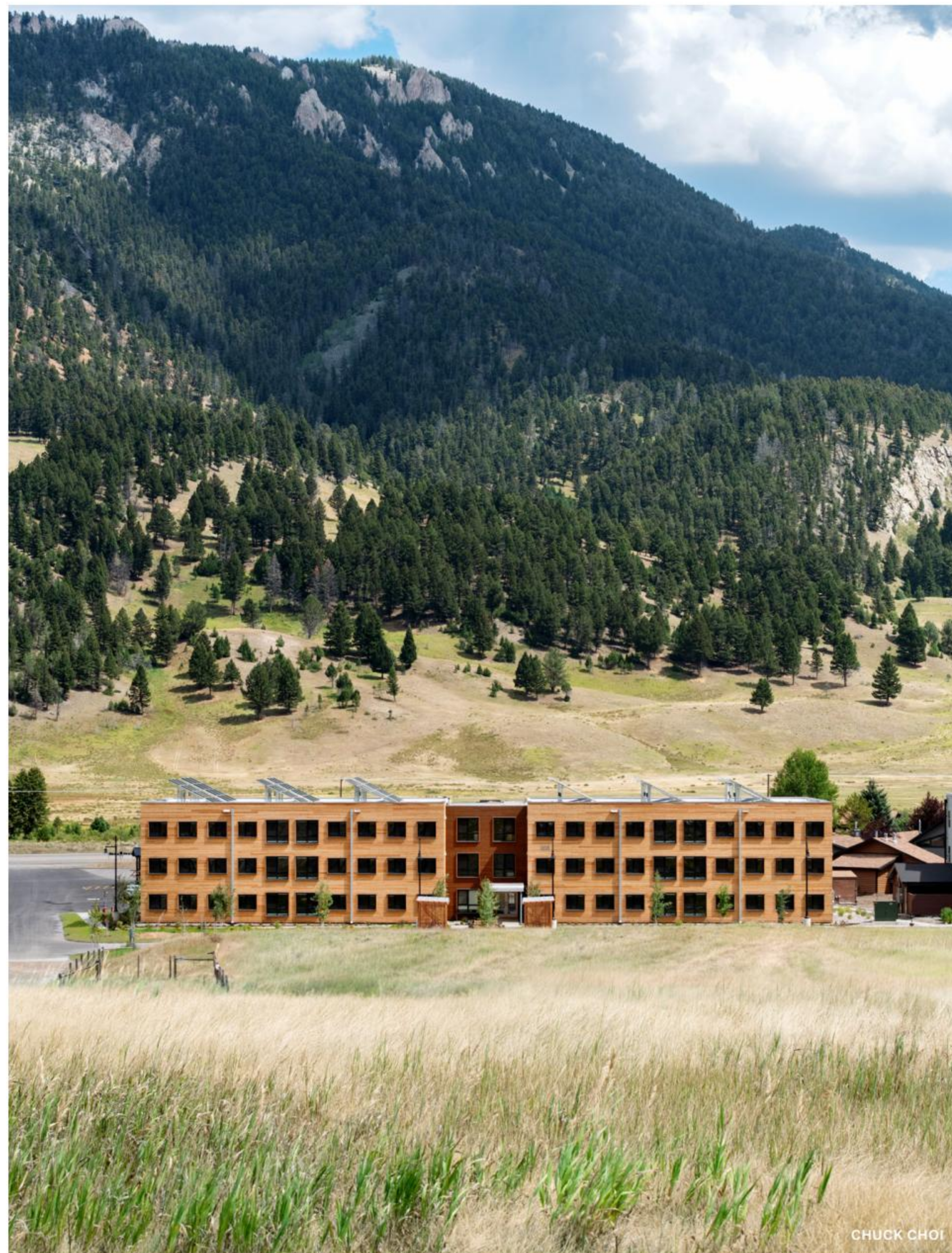
In Big Sky, Montana, Peter Rose + Partners designed the nation's first modular mass-timber structure, a 32,000-square-foot building for temporary workers.
