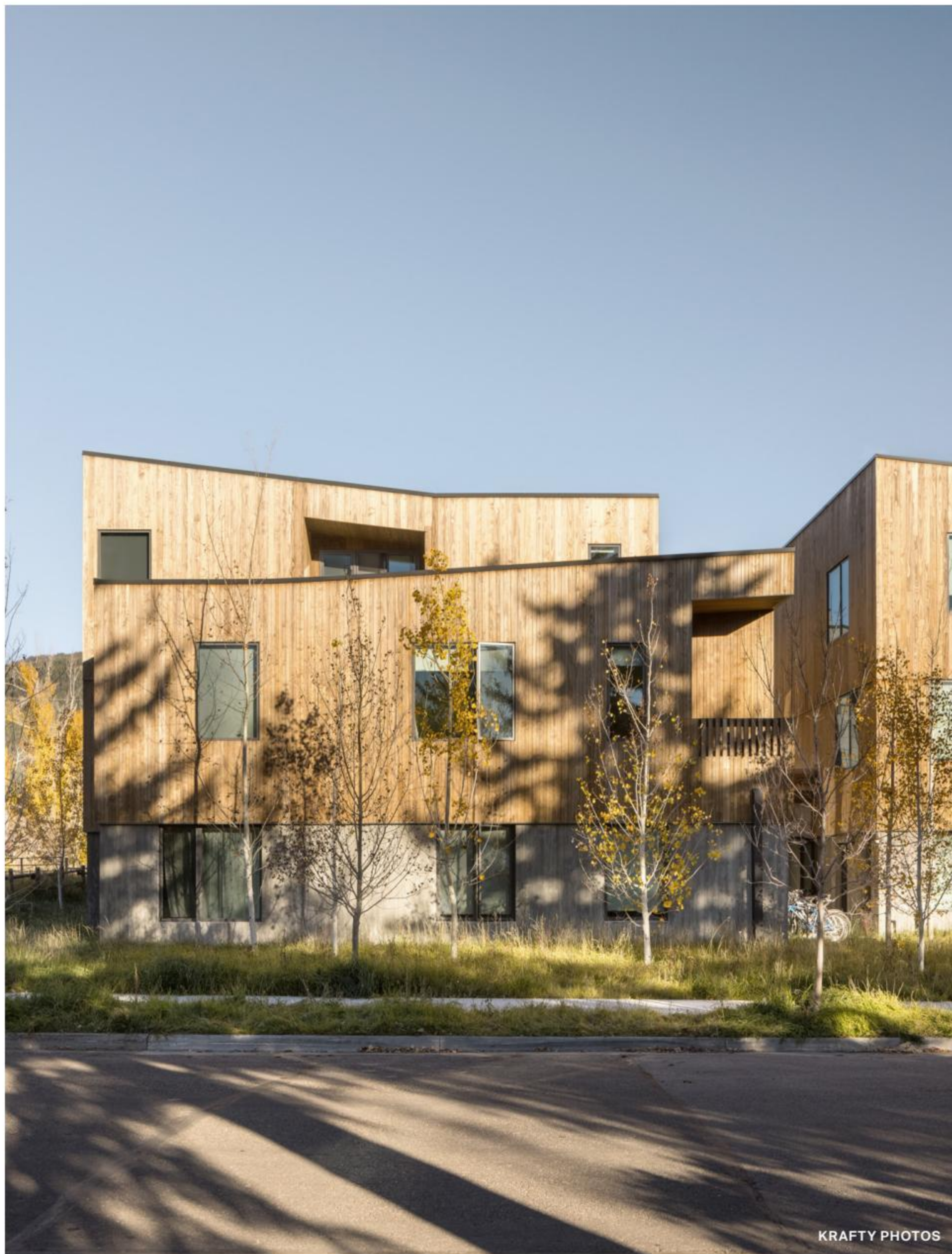
A 20-unit development of workforce housing by Merge Architects in Jackson boasts light-filled one- and two-bedroom apartments with private balconies and shared courtyards.
