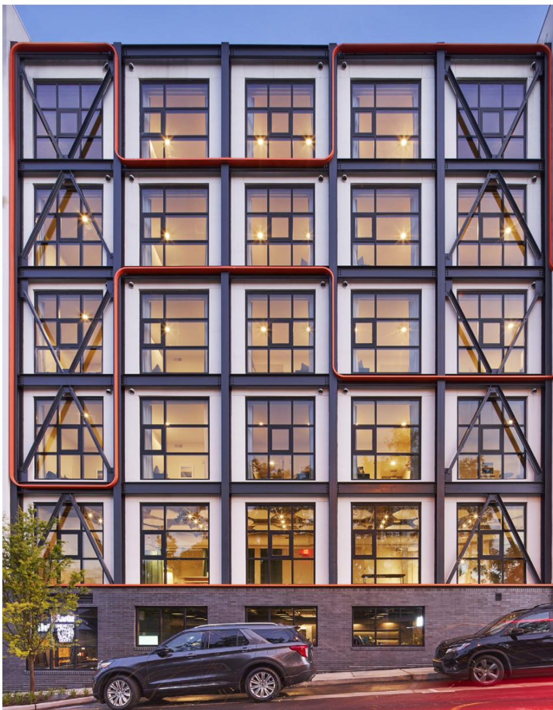
Corey Gaffer, Gayle Babcock/Courtesy Architectural Imageworks
