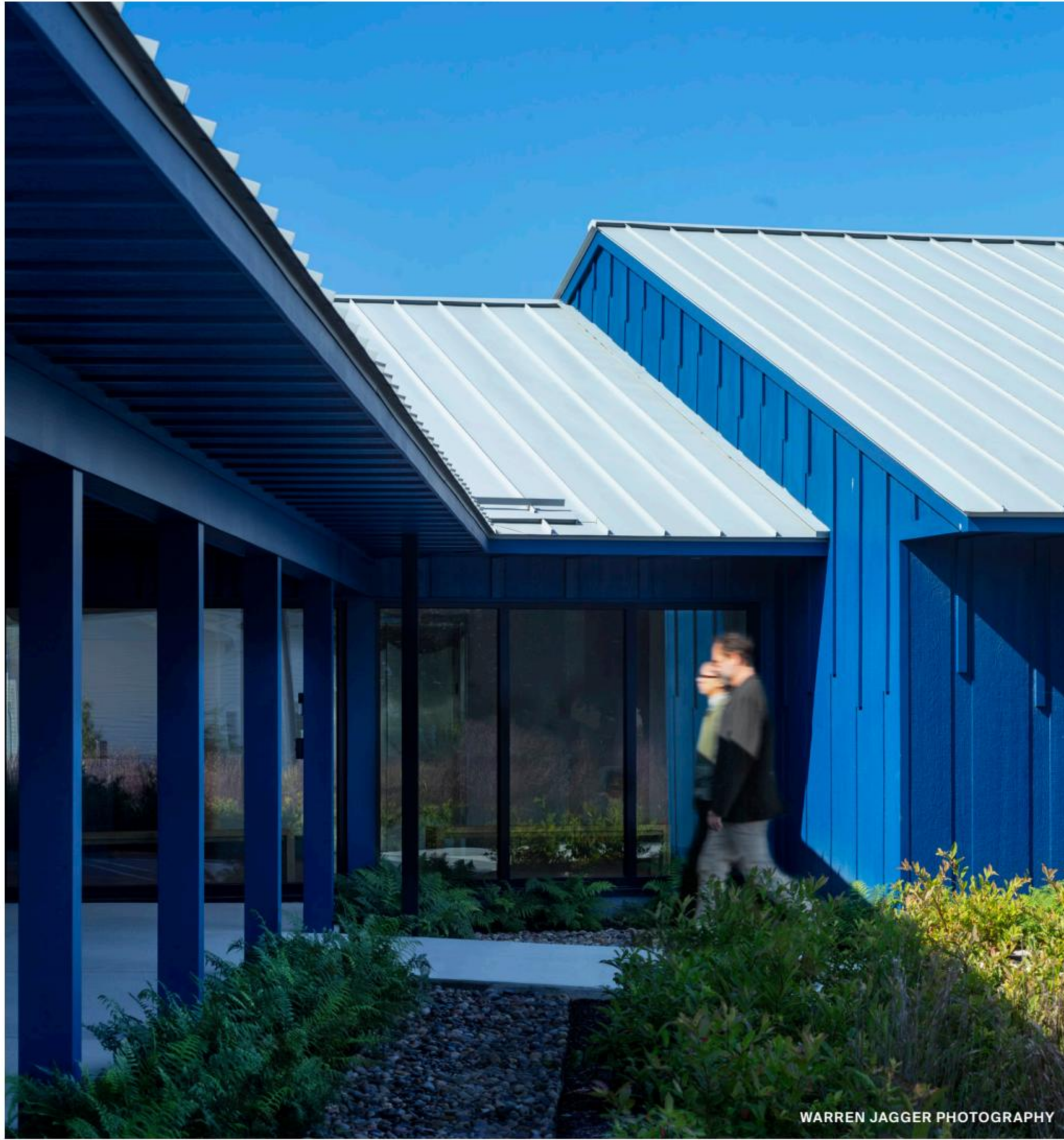
The exterior of the Westerly Museum of American Impressionism is clad in a new composite wood sheathing whose blue color is designed to make the meadow pop.
