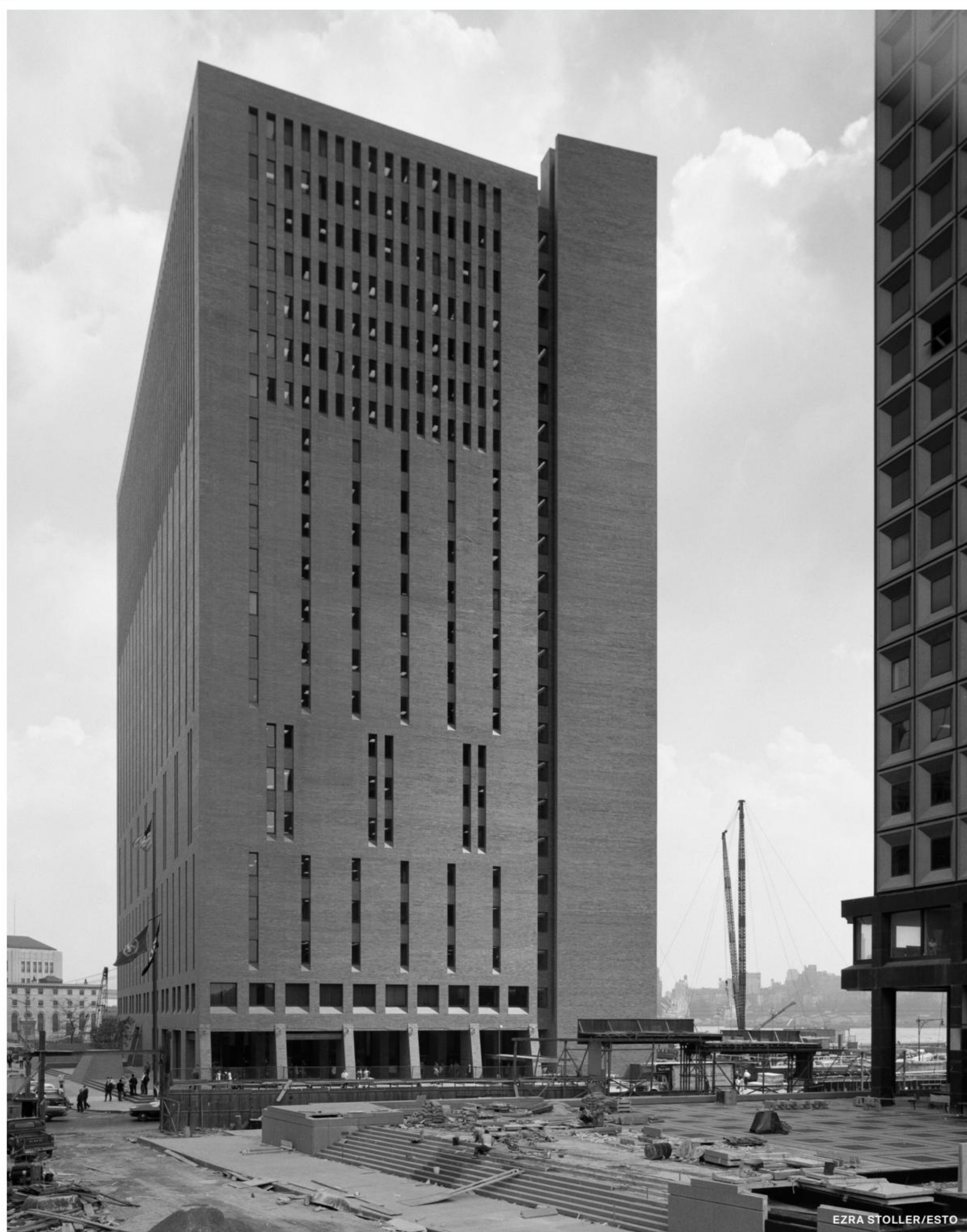
The office building at 25 Water Street was recently converted into apartments by CetraRuddy.
