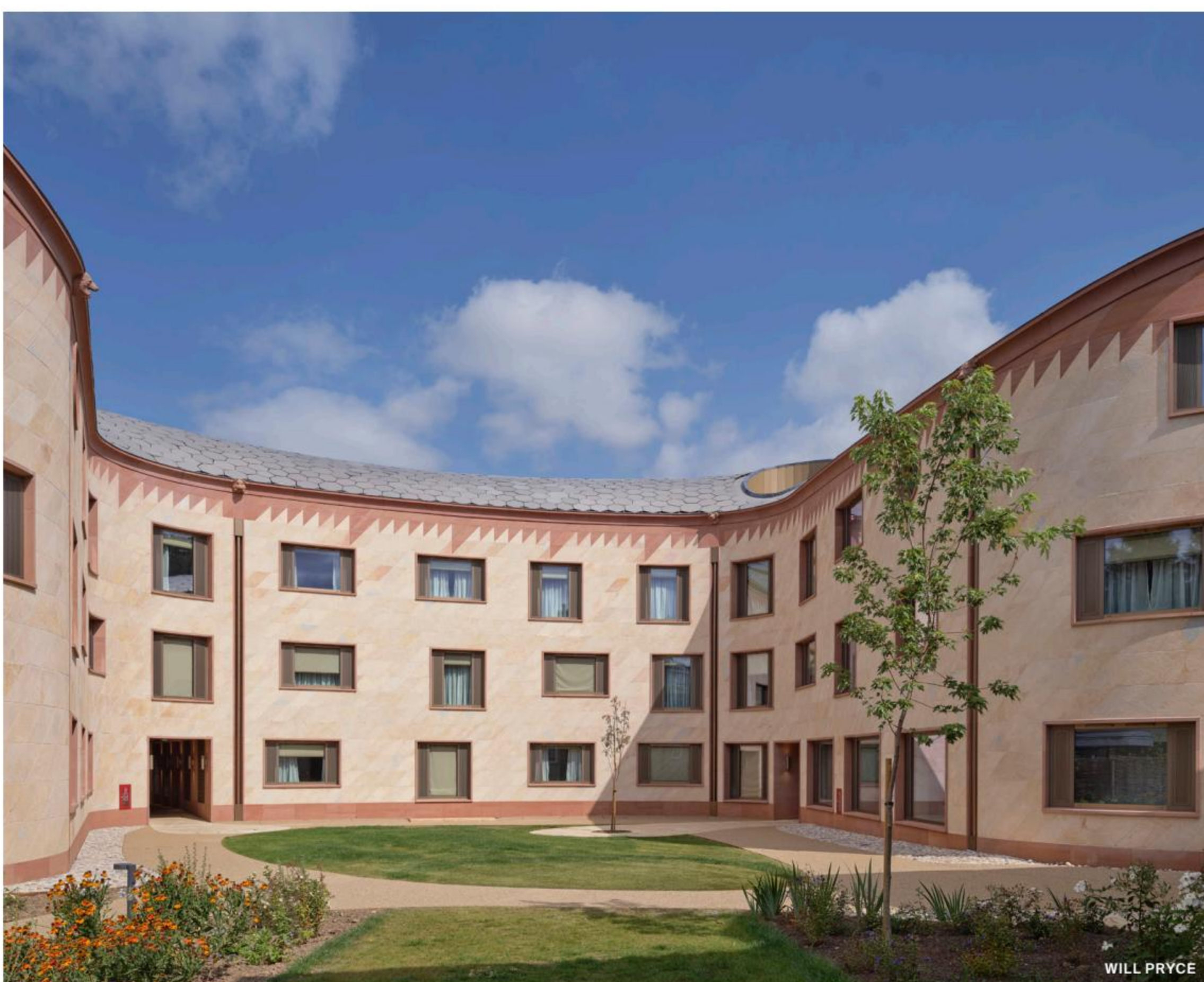
Flames of red appear in the diamond formation of the stone blocks that pick up on the pink Cumbrian sandstone plinth and jagged cornice.
