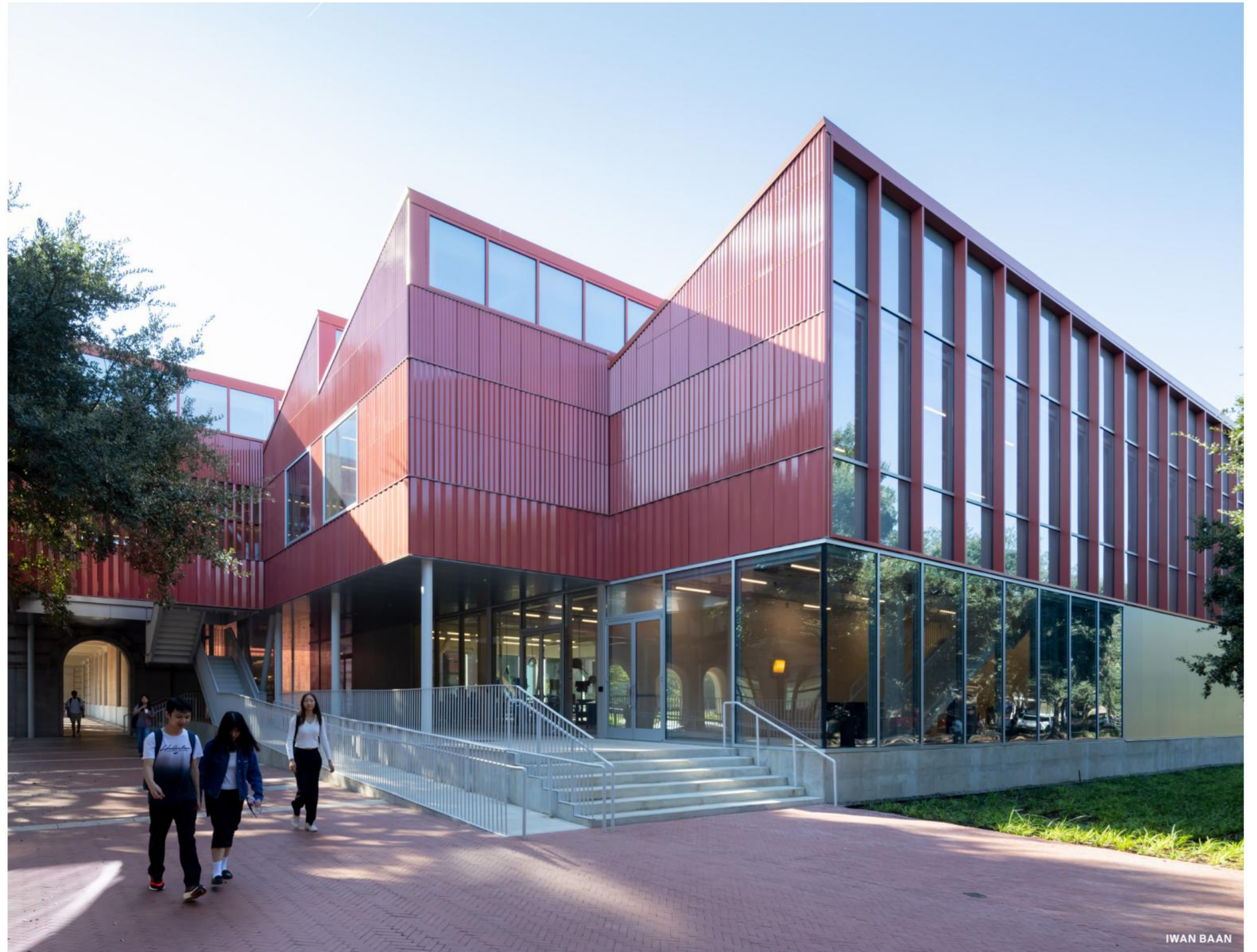
Above: The young Swiss architecture firm Karamuk Kuo has created a “marvelous enigma” with Cannady Hall at Rice University. Its deceptive facade appears to be made of simple red metal panels but is instead glazed terra-cotta battens.
