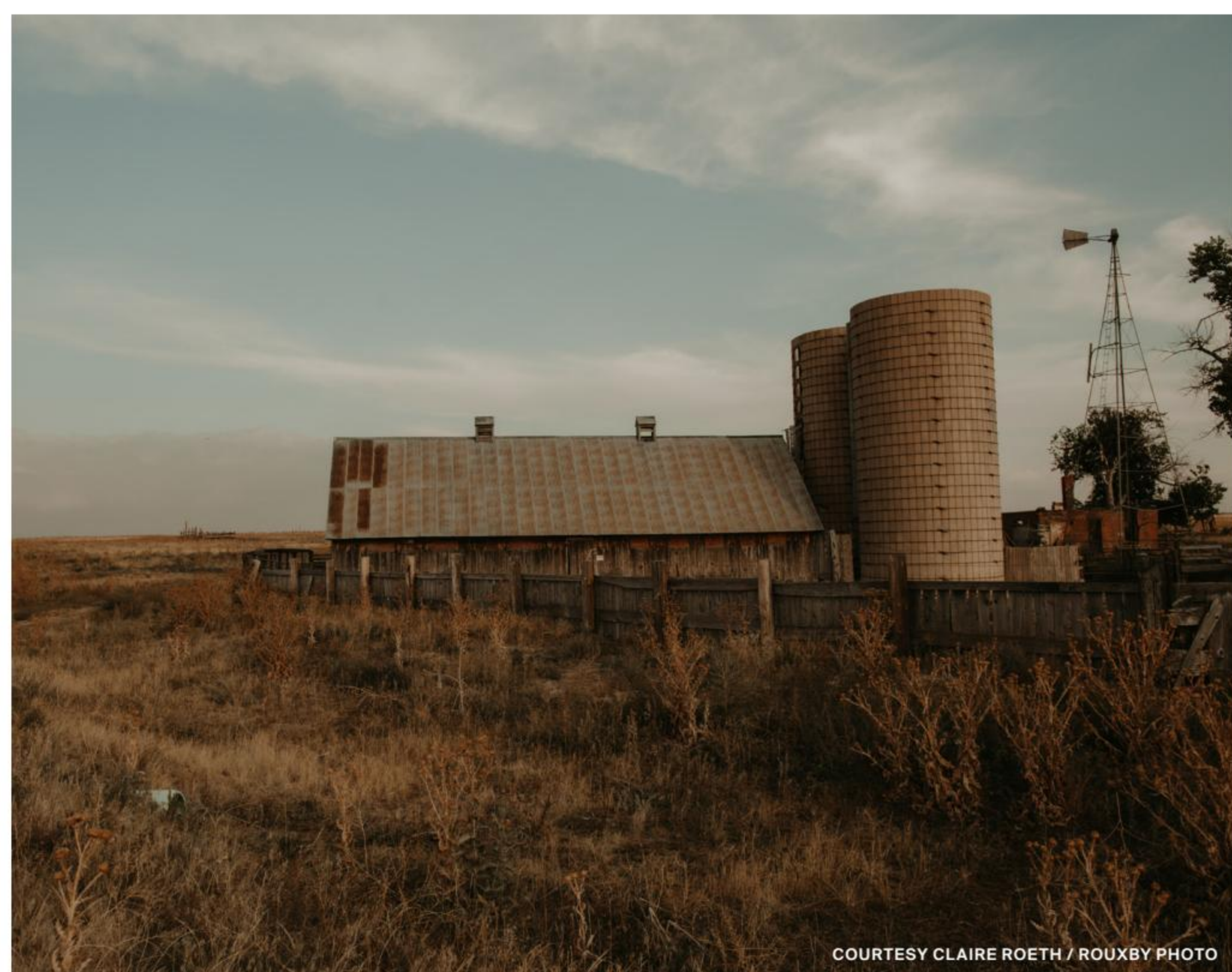
Top: Superbloom designed 1881 Farm Park in Denver with an eye to the past and the future, incorporating existing structures and creating a landscape that will evolve; the site will feature a market and seasonal restaurant. Above: A repurposed barn at 1881 Farm Park, also visible in the rendering at top.
