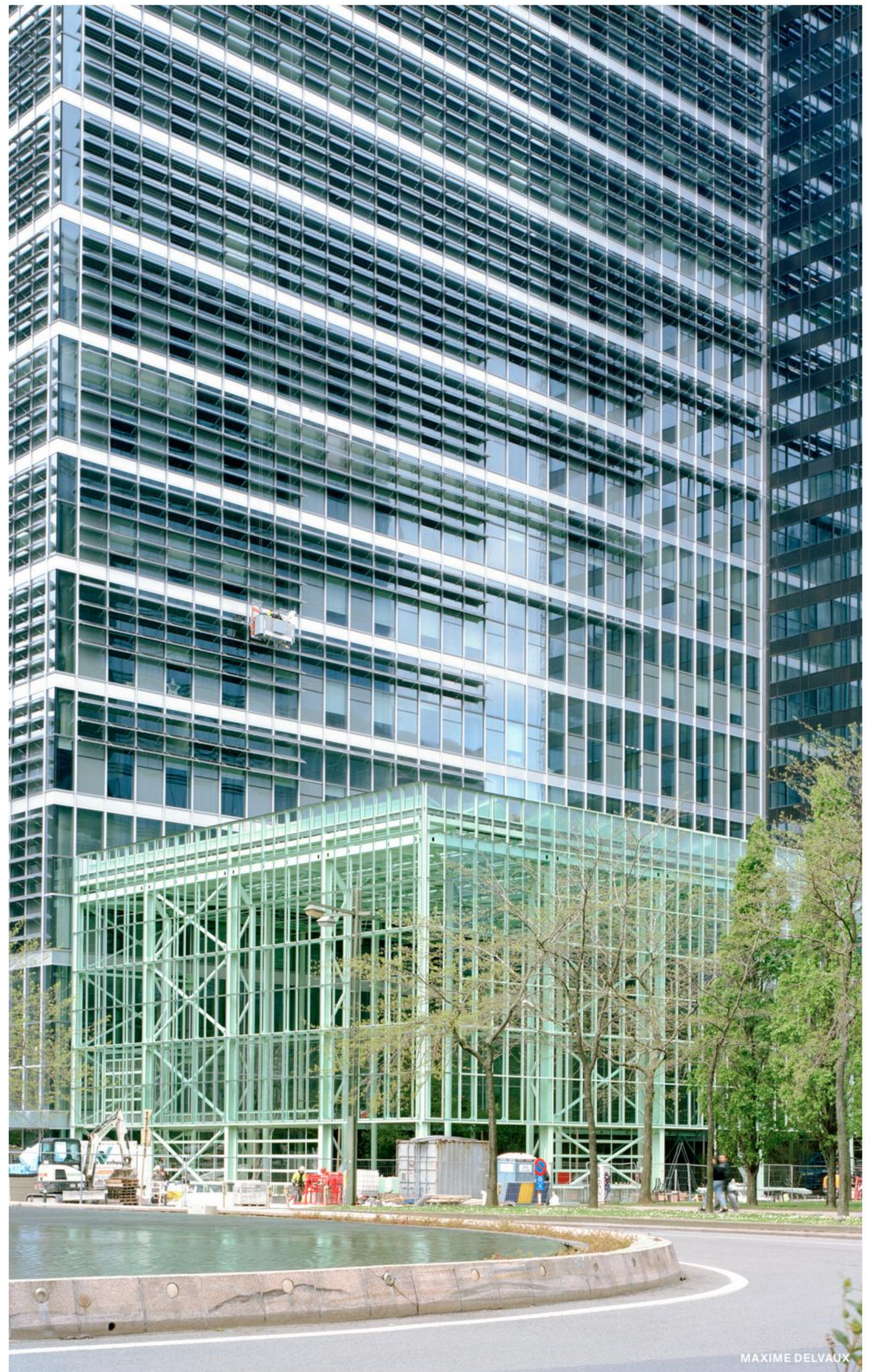
ZIN, seen while under construction. 51N4E claims it retained 60 percent of the original WTC by weight, while others argue that the realities of its construction—new floor plates and facades—constitute a form of adaptive reuse—washing.
