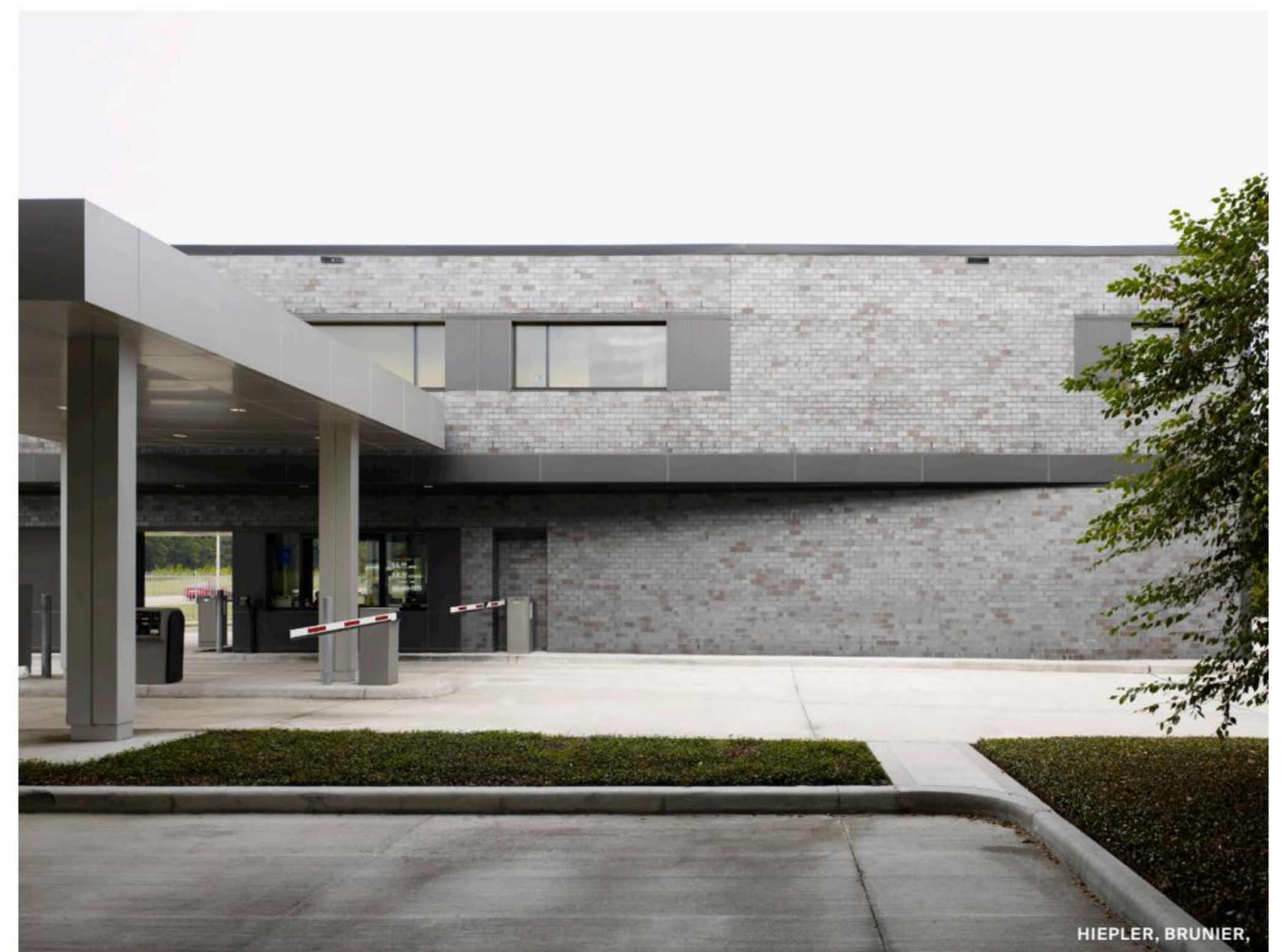
The second floor of the administration building cantilevers slightly over the ground floor as it is pinched, allowing for two lanes of car traffic in and out of the complex. This detail makes the narrow building even thinner, as seen in the plan and section above.
