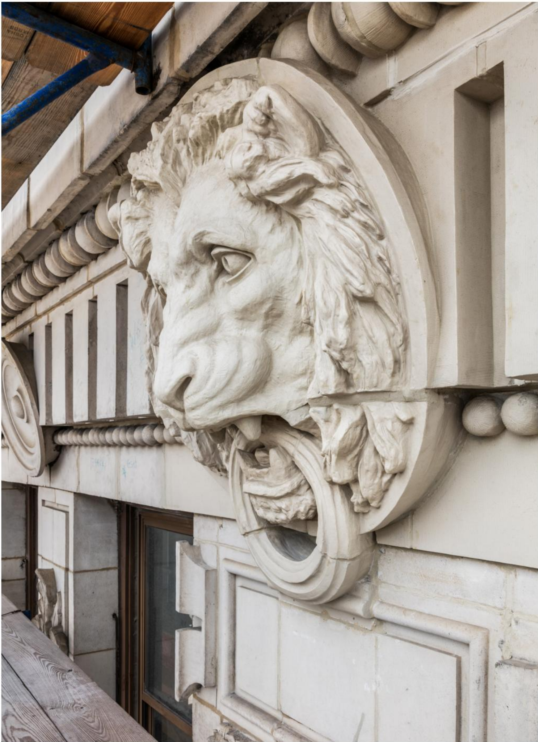
Christopher Payne's photographic project extended beyond the Gladding, McBean factory and onto construction sites like New York's Flatiron Building, shown here, where new hand-molded terra-cotta pieces were installed.
