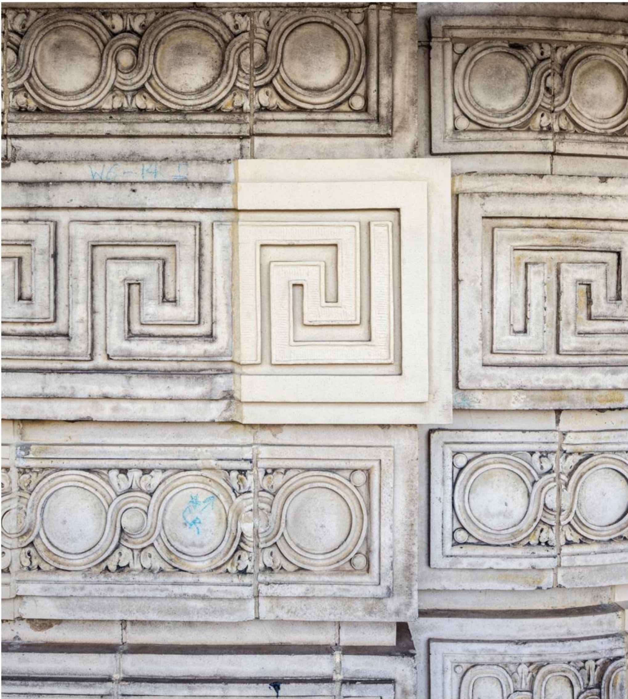
Christopher Payne's photographic project extended beyond the Gladding, McBean factory and onto construction sites like New York's Flatiron Building, shown here, where new hand-molded terra-cotta pieces were installed.
