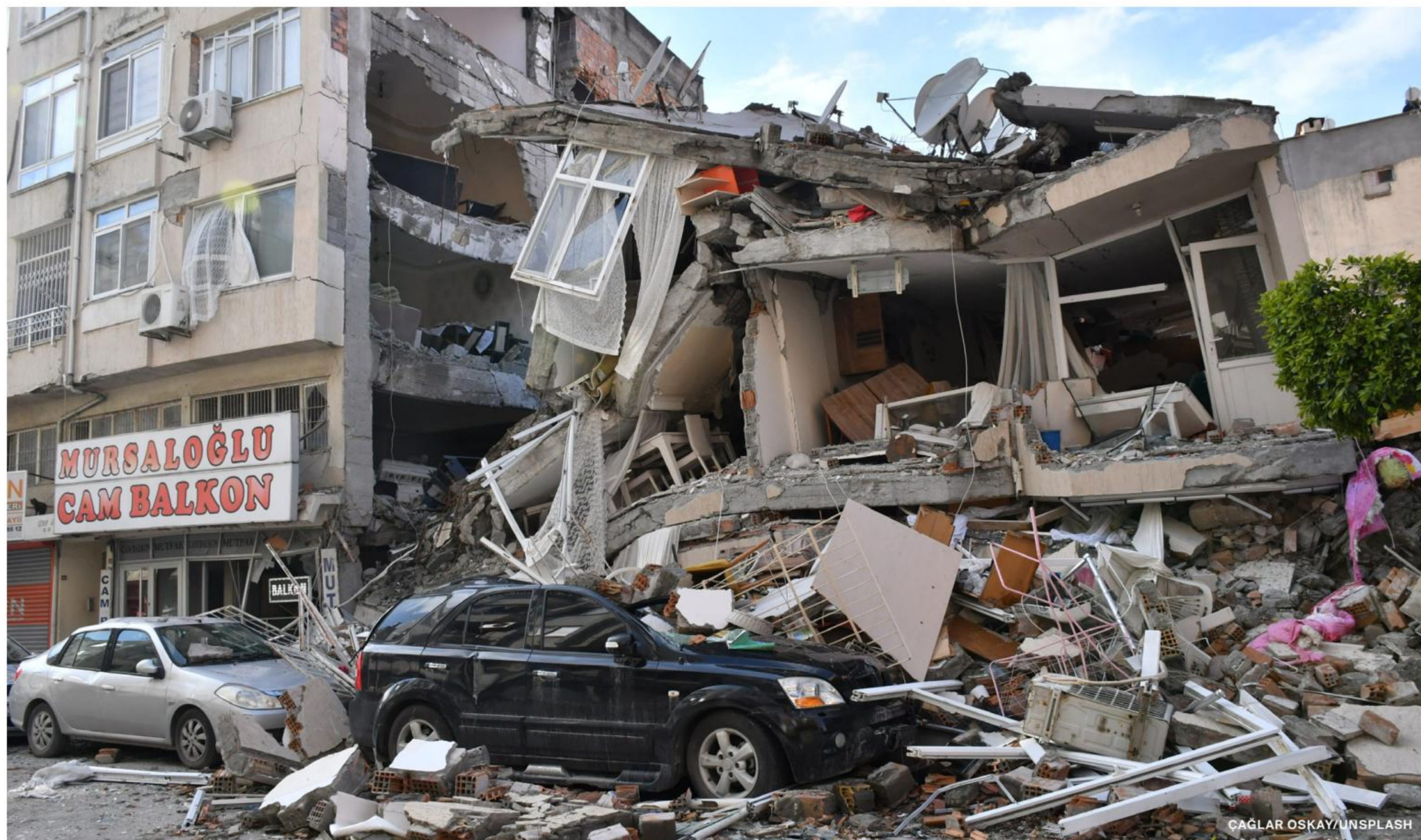
Earthquake damage in Iskenderun, a city along the Mediterranean Sea in Turkey's Hatay province
