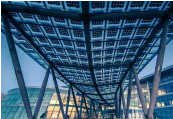
SOLARVOLT Building Integrated Photovoltaic (BIPV) Modules Vitro Architectural Glass
