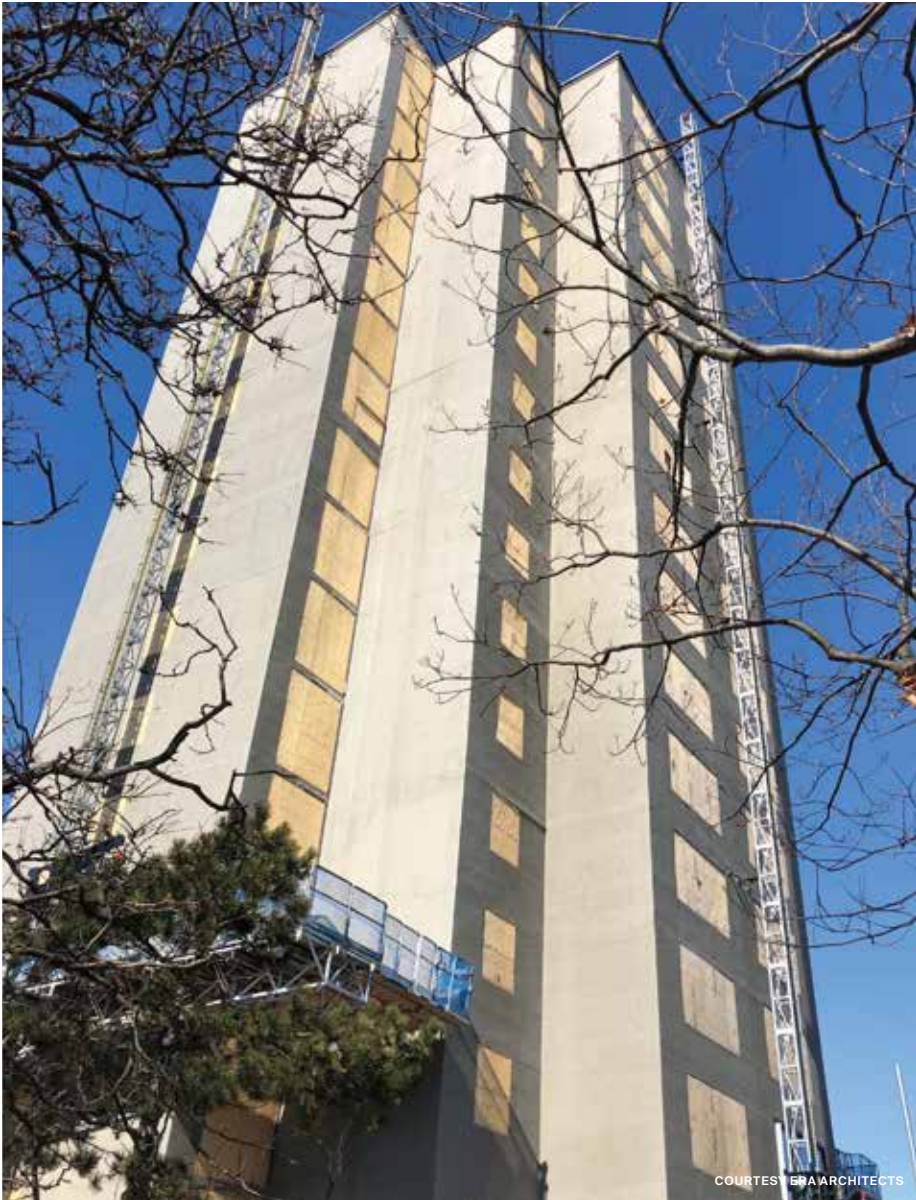
The entire facade was treated with a fluid applied air barrier and a layer of fiberglass insulation.
