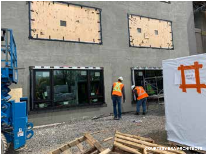
The windows bays were slightly expanded and replaced with triple-glazed units.
