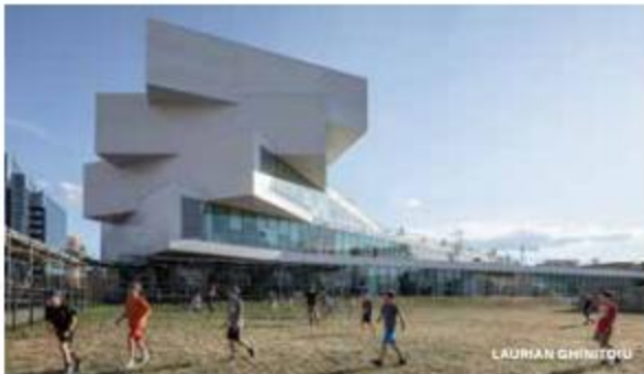
The Heights Building in Arlington, Texas, designed by BIG, features a cascading facade with YKK's unitized wall system.
