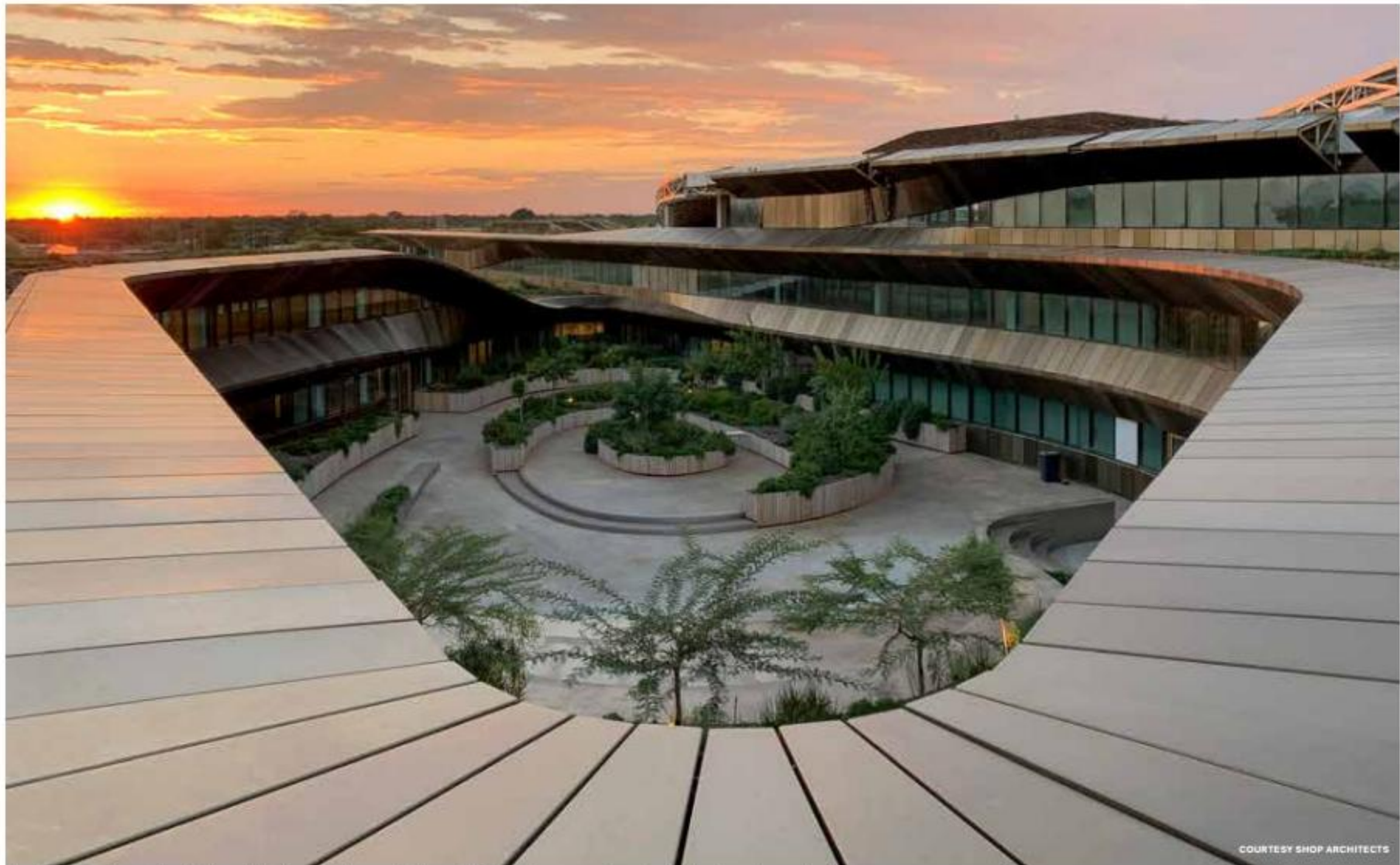
The Botswana Innovation Hub's undulating canopies echo the region's landscape, and courtyards break up the project's mass.
