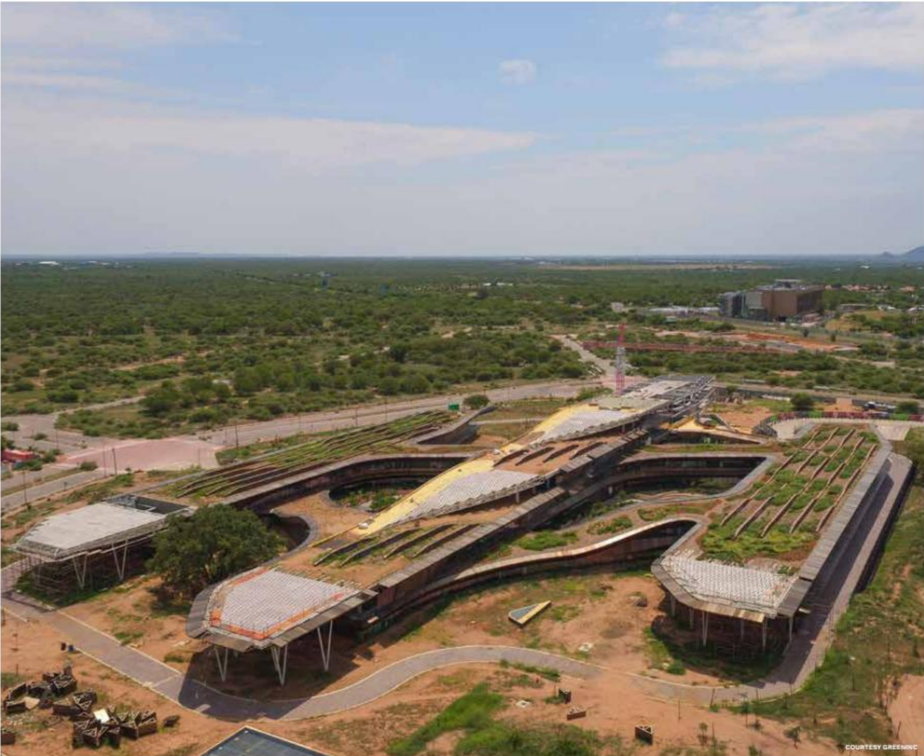
SHoP Architects developed the facade system's design as a customized kit-of-parts. The pieces were fabricated in South Africa, shipped hundreds of miles north, and assembled and installed on site. Every step of the process was digitally tracked and monitored from New York.
