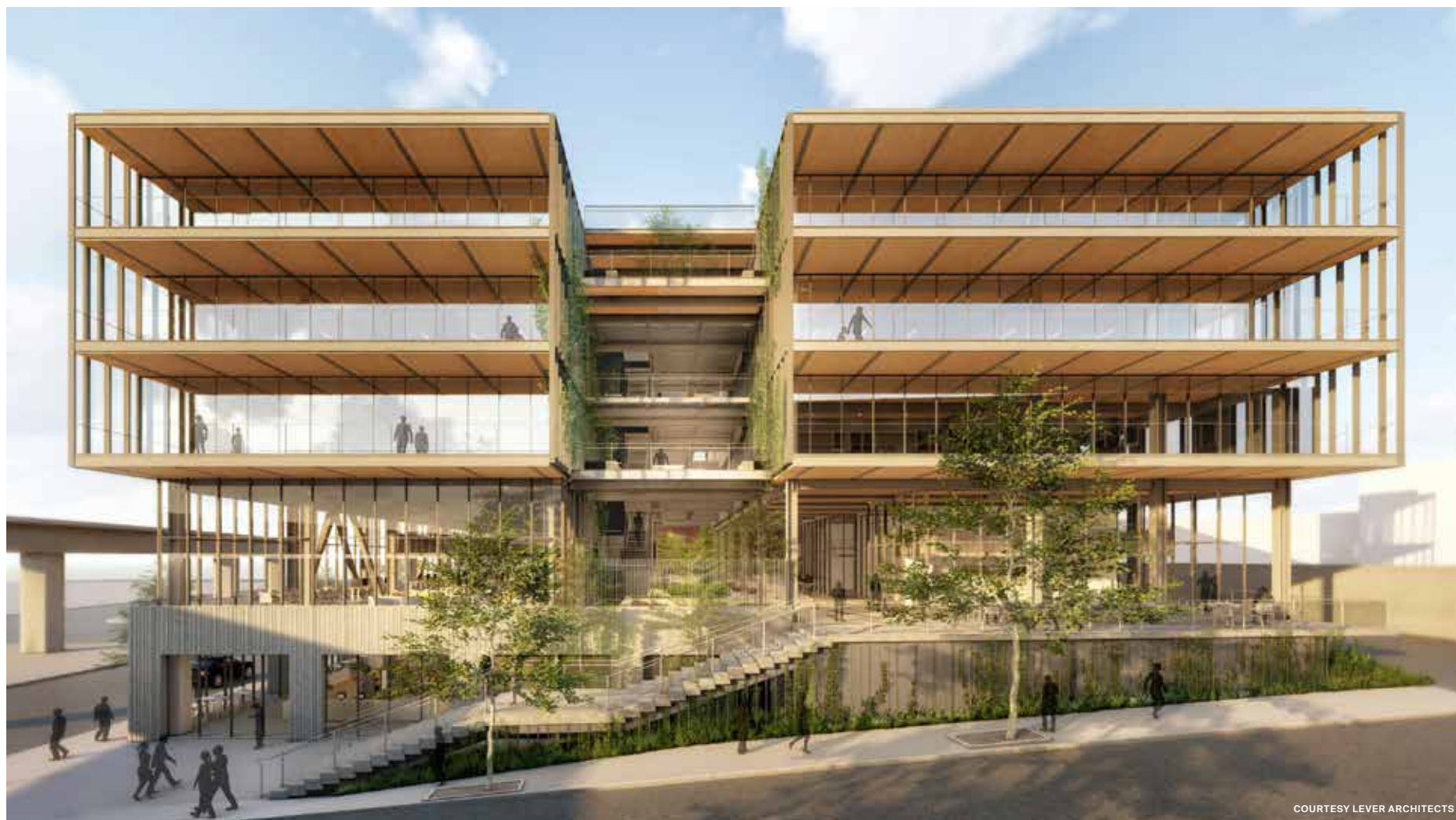
843 N Spring Street in Los Angeles by LEVER, shown in a rendering here, has a hybrid structural system that combines a CLT floor system with exposed steel columns and beams.
