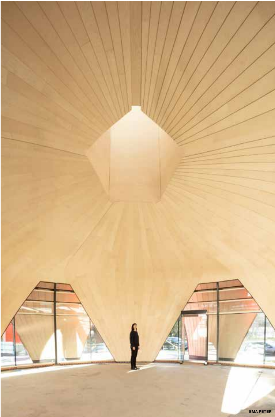
Above: The interior of the pavilion is treated with narrow strips of birch plywood. A central oculus and glazing bays provide ample daylight.
