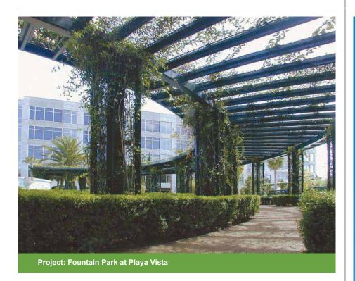
greenscreen® panels can be tapered or angled in conjunction with steel by others to create a walkway of dappled shade.
