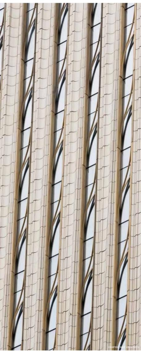
$SHoP\ Architects\ developed\ a\ wavelike\ format\ for\ the\ terra-cotta\ panels\ using\ parametric\ design.$
