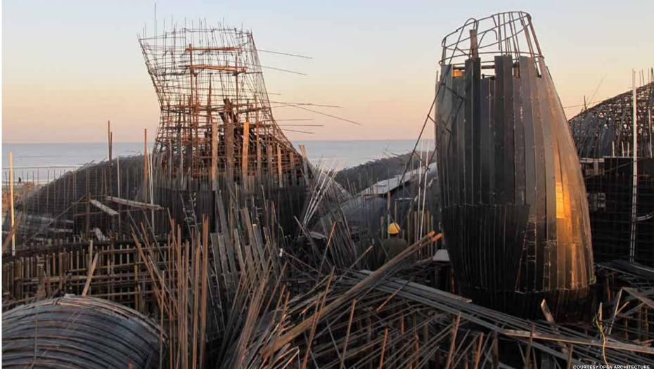
**Top:** OPEN Architecture changed their initial plans to plaster over the concrete walls in order to maintain what founding partner Li Hu calls "the raw but truthful quality of the concrete texture." **Above:** The sculptural formwork was made almost entirely from narrow strips of wood.
