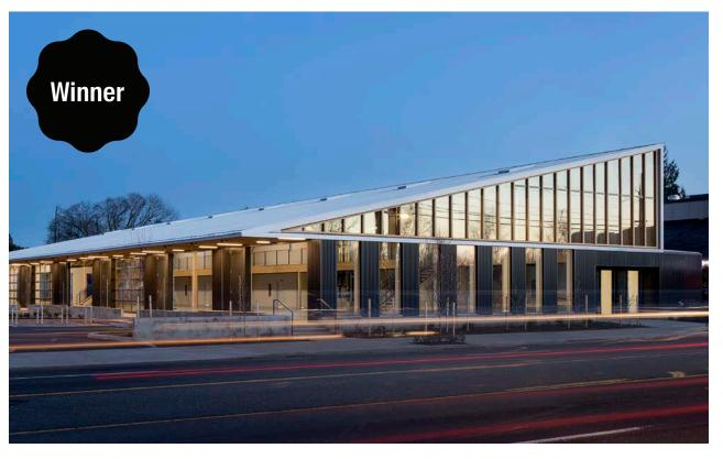
FLEX is a 19,000-square-foot building that can be adapted for various commercial uses. LEVER Architecture developed the design based on an industrial typology that incorporates mass timber structural elements, a distinctive angular frame, and interior mezzanines. The large, 200-by-95-foot open floor plate is divisible into eight 24-foot structural bays, allowing the building to be partitioned for diverse tenants—from a restau-
