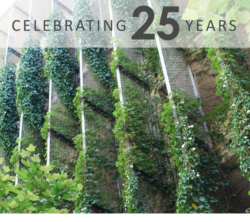
The benefits of three-dimensional, welded steel wire construction are evident in the capabilities of greenscreen® trellis panels in many applications. With appropriate plant material, the greenscreen® system offers the potential of both ecosystem services available from a green facade and unique aesthetic benefits to a building, its landscape environment, and its users.
