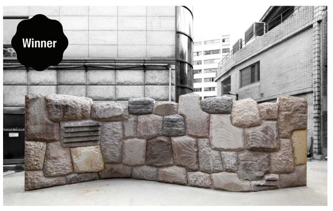
By translating an ancient method of masonry into a digital procedure, Matter Design developed Cyclopean Cannibalism as a sustainable alternative to the standard practice of landfilling demolition debris. This project illustrates how the carcasses of previous buildings could be reused as a new material. To do this, rubble is scanned and input into a digital algorithm that sorts random shapes. Each stonelike component
