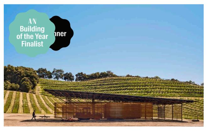
Located in West Paso Robles, California, this unassuming agricultural storage facility was constructed using salvaged oil drill stem pipes, WT steel, Douglas Fir plywood, and perforated metal screen panels. Sliding barn doors are clad in a tube steel frame forged from remnants of the winery's shoring wall. The pole barn sits sentry as the first structure near the entry of the 50-acre James Berry Vineyard. The building's
