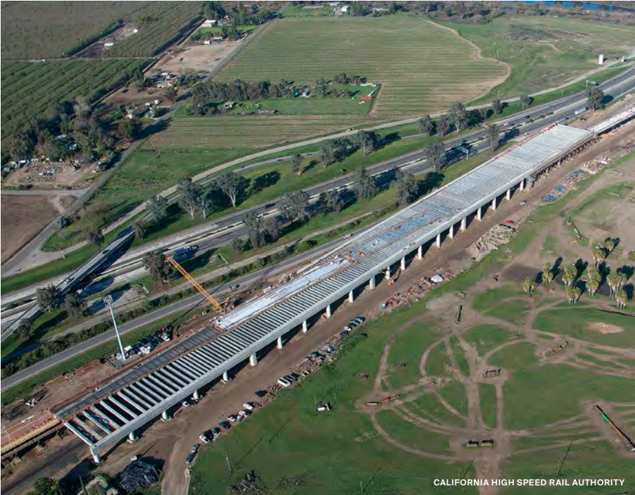
The California High Speed Rail Authority is deep into construction on the first leg of what will be a $100 billion bullet train. Above: Crews work on a section of the San Joaquin River Viaduct & Pergola in Fresno that will allow the rail line to fly above existing highways and city streets.
