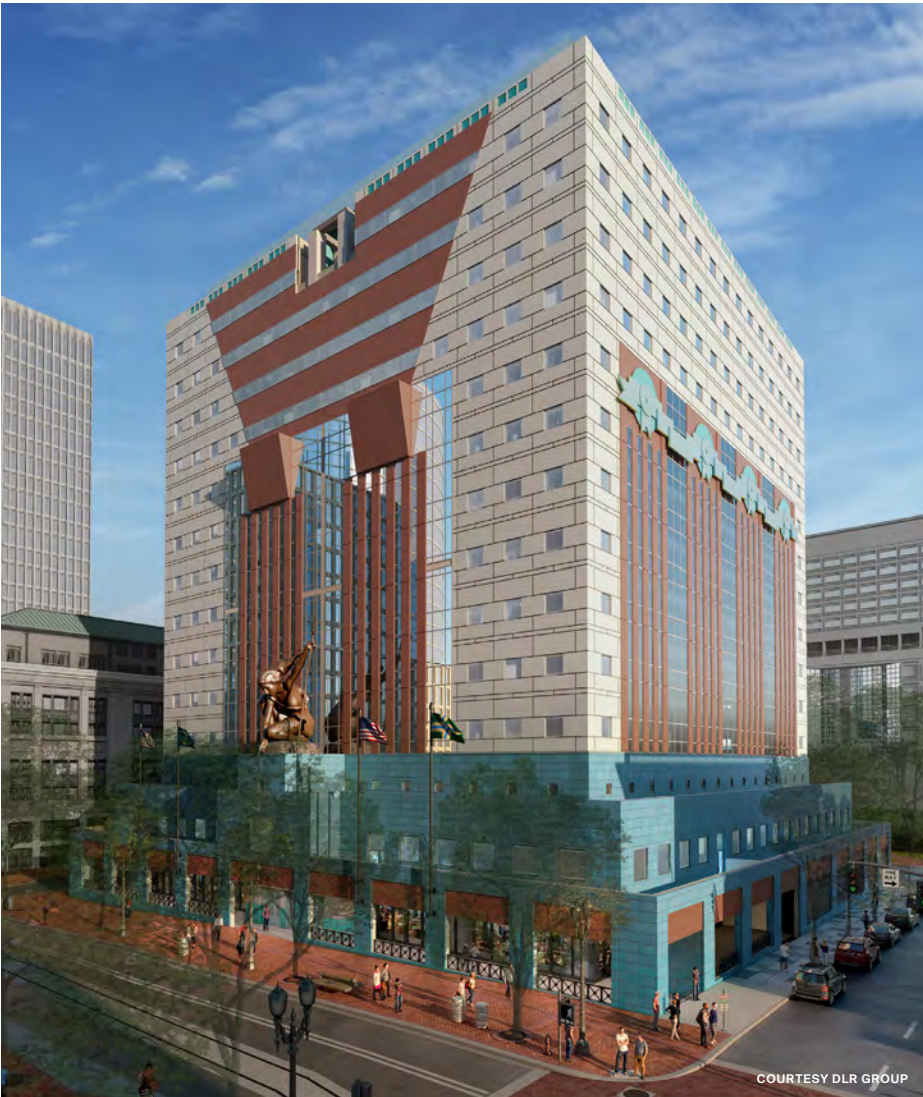
DLR Group is pushing ahead on renovations to Michael Graves's iconic Portland Building that aim to reskin the iconic postmodern office tower with a unitized aluminum rainscreen.
