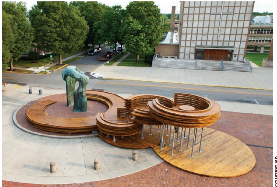
With few precedents to follow, the hardwood CLT Conversation Plinth in Columbus, Indiana, needed to be engineered from the ground up using the latest digital stress models.
