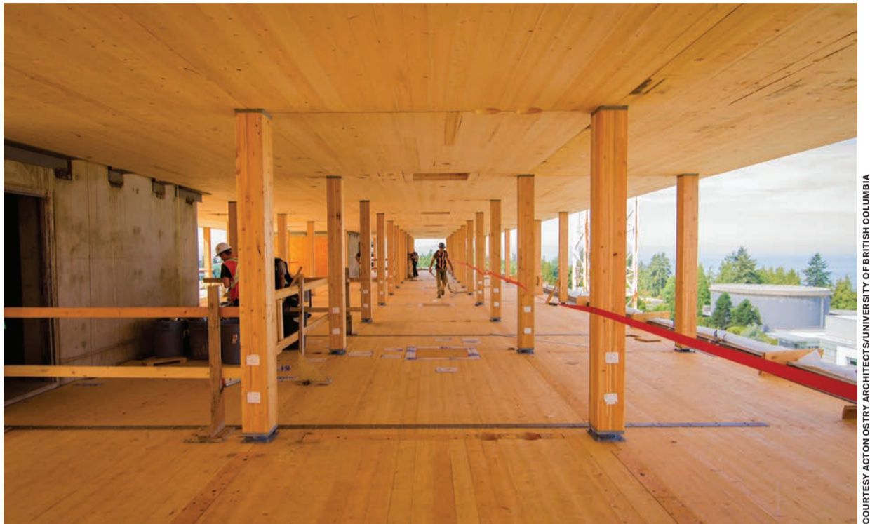
With their 18-story Brock Commons project, Acton Ostry Architects supplemented the mass timber walls, columns, and floors with a concrete core in order to allow for a taller, more rigid structure.
