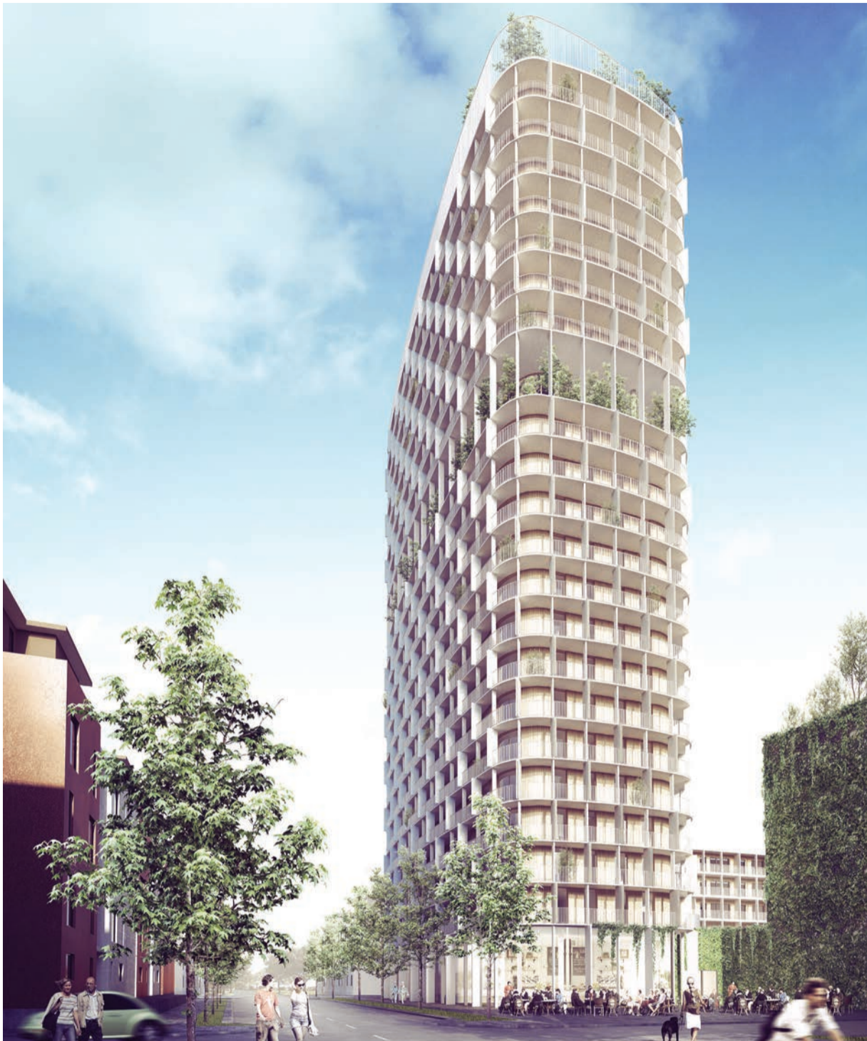
A new 23-story housing tower by C.F. Møller features seven levels of mass timber construction and a roof terrace. The mass timber floors sit above 15 levels of traditional concrete construction.
