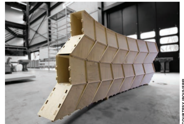
The pavilion's spanning arches are built from piecemeal CLT elements that snap together.
